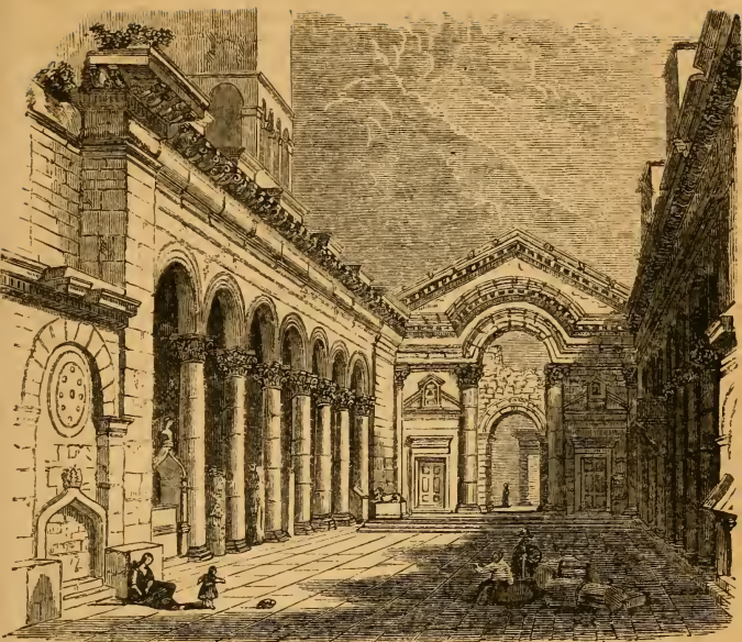
The Court-yard of Diocletian's Palace at Spalatro.
