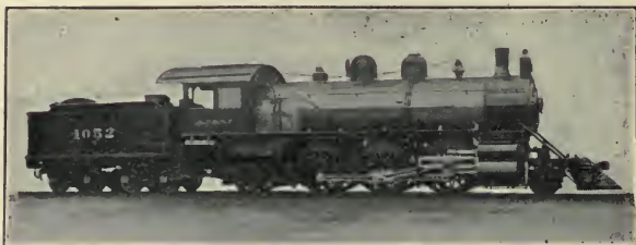
THE MOGUL TYPE OF COMPOUND FREIGHT-ENGINE, BALDWIN LOCOMOTIVE WORKS.
