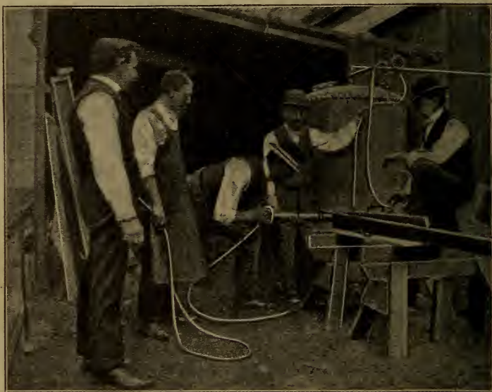
FIG. 52.—THE BOYER HAMMER DRIVING 1-INCH RIVETS.
