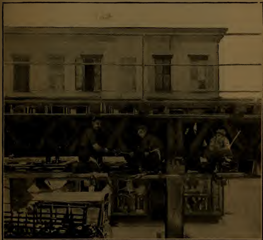
FIG. 368—DRILLING AND RIVETING ELEVATED R. R. STRUCTURE.
