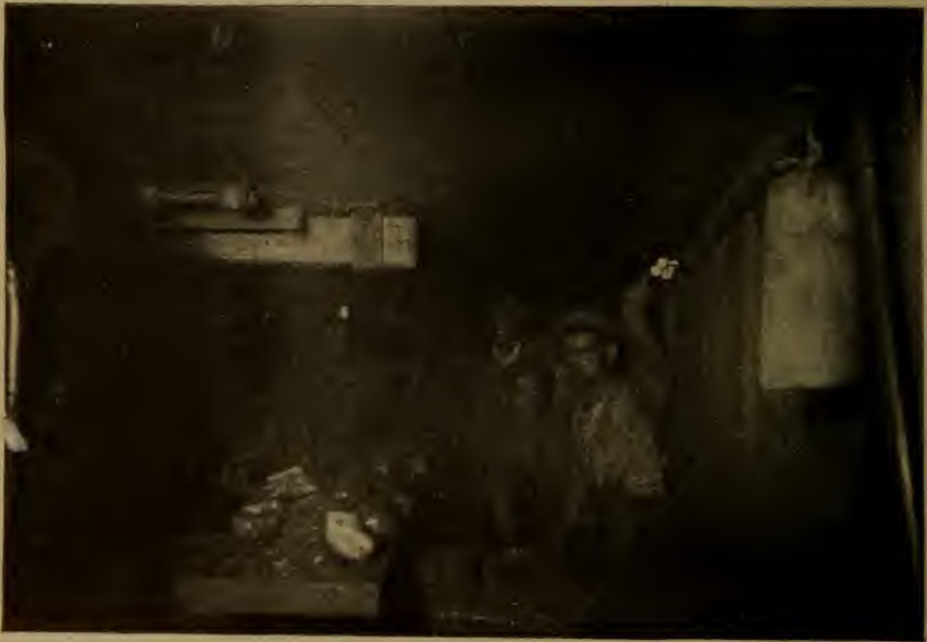
FIG. 433—FLASHLIGHT IN CAISSON.
