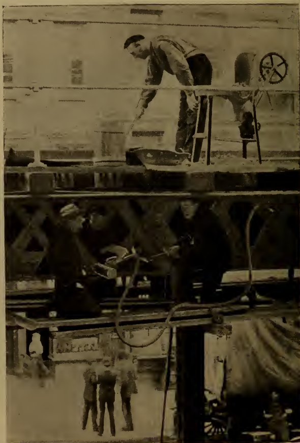
FIG. 369—RIVETING WITH YOKE RIVETER.
