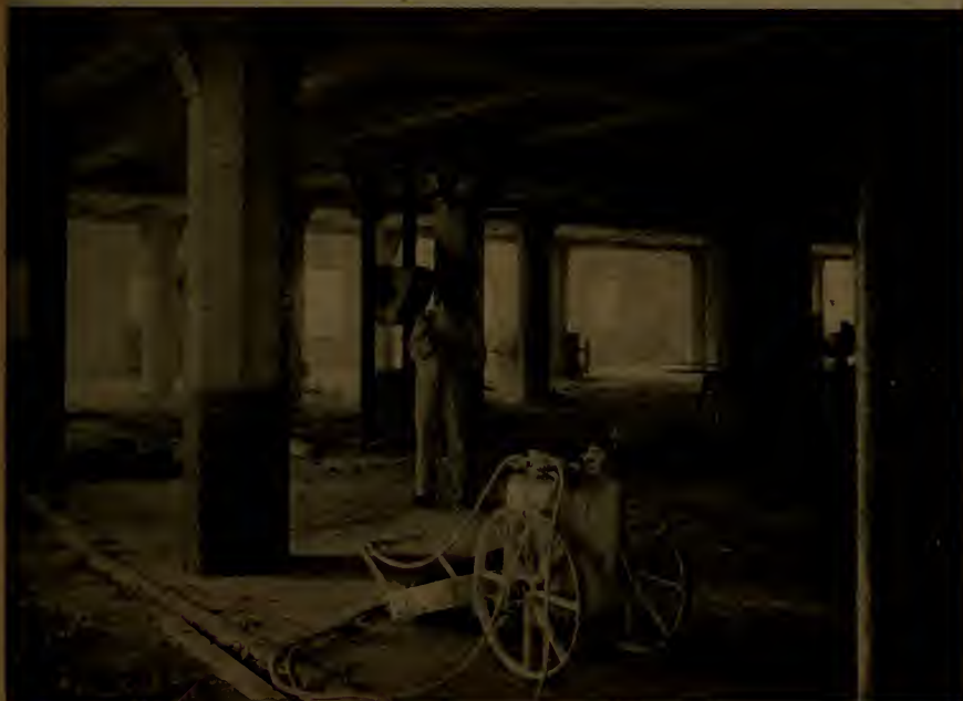
FIG. 326.—PAINTING ARBUCKLE SUGAR REFINERY BY THE BRYCE PNEUMATIC PAINT MACHINE.
