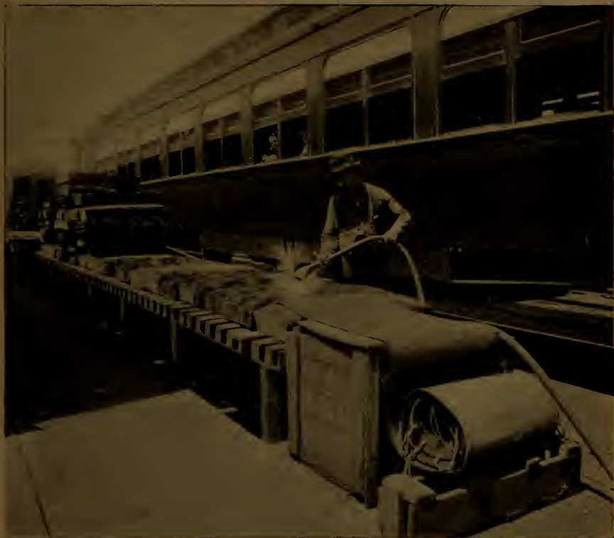
FIG. 474—CLEANING CAR SEATS WITH AIR.
