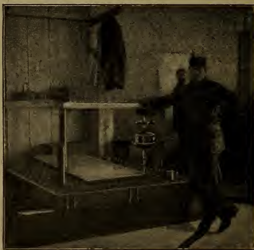
FIG. 478—PNEUMATIC DRILL, IN SHIP-YARD WORK.
