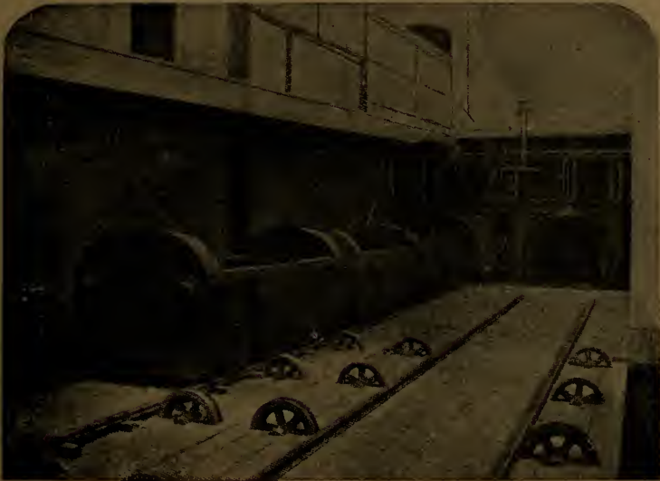
FIG. 182—TRAIN OF CARS, HOLBORN STATION.
