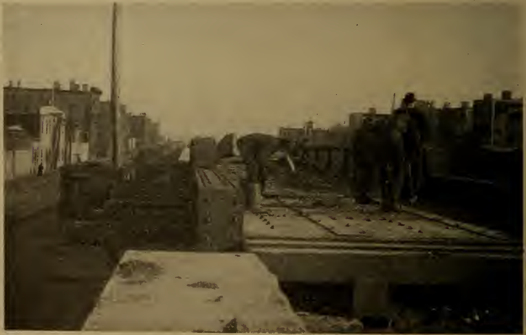
FIG. 376—RIVETING ON BRIDGE ERIE R. R. ELEVATION. POWER OBTAINED FROM GASOLINE AIR COMPRESSOR IN BOX CAR TO THE LEFT.
