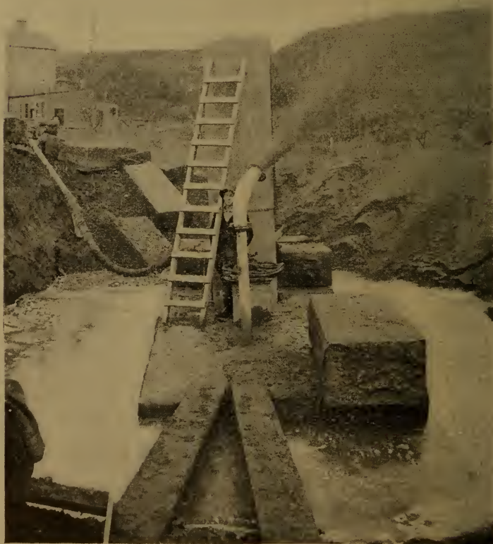
FIG. 432—CAISSON NO. 3 BLOWING SAND.
