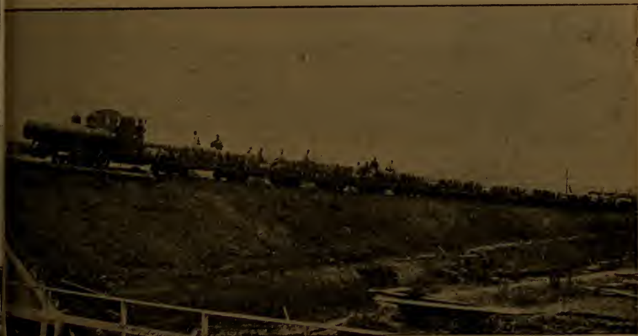
FIG. 176—COTTON TRAIN AT PORT CHALMETTE—COMPRESSED AIR LOCOMOTIVE.
