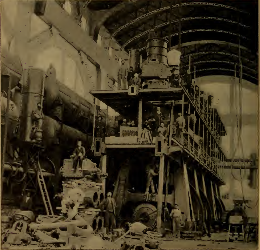
FIG. 63.—AIR COMPRESSORS AND AIR STORAGE RESERVOIRS.
