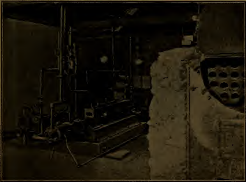
FIG. 94.—HIGH RANGE AIR COMPRESSOR IN SERVICE.
