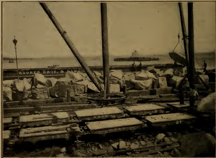
FIG. 314.—THE USE OF COMPRESSED AIR IN BUILDING THE DELAWARE BREAKWATER.
