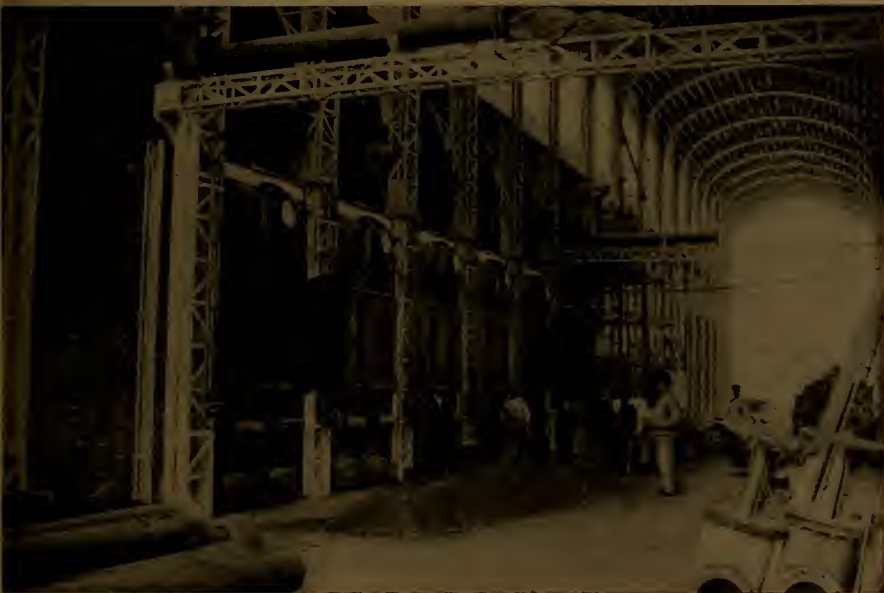
FIG. 62.—BOILER ROOM OF THE PARIS PLANT.
