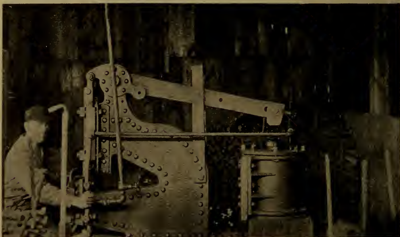
FIG. 303—PNEUMATIC SCRAP SHEARS.
