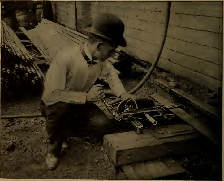
FIG. 349.—PNEUMATIC RAIL DRILLER.
