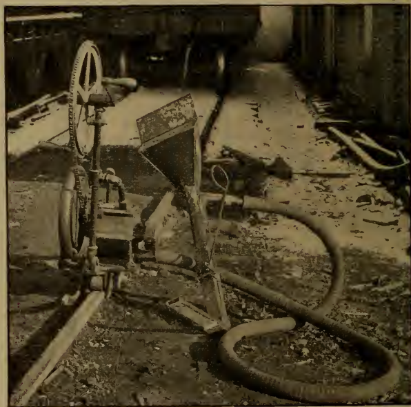
FIG. 440—MACHINE FOR SURFACING RAILROAD TRACK BY MEANS OF COMPRESSED AIR.
