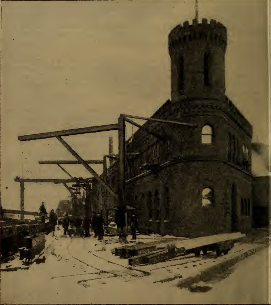
FIG. 293.—UNLOADING CARS WITH AIR HOISTS.
