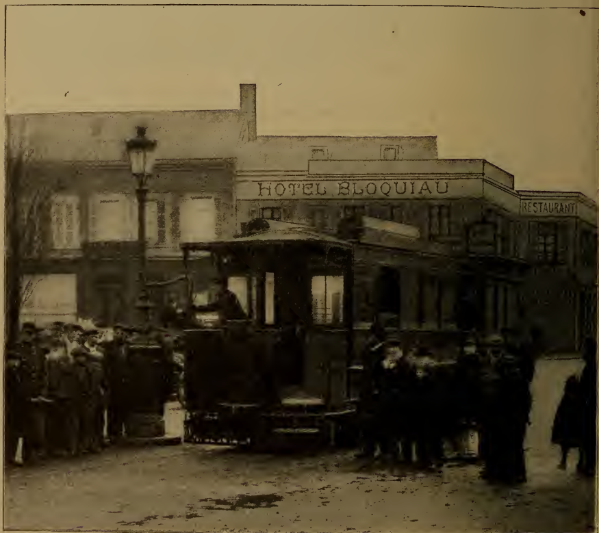
FIG. 170—COMPRESSED AIR TRACTION IN PARIS. CHARGING STATION ON A PARIS TRAMWAY.
