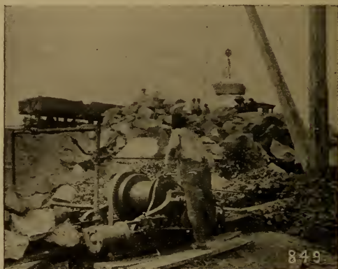
FIG. 324.—HOISTING A 3 TON ROCK BY AIR POWER.
