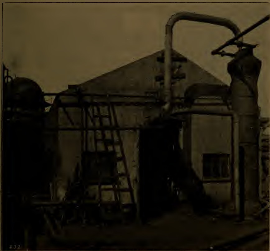
FIG. 117.—REHEATING AT PUMPS.
