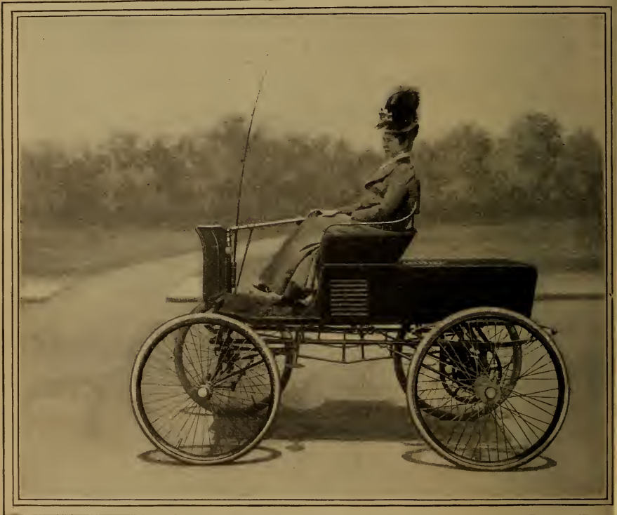
FIG. 168—THIS AUTOMOBILE IS OPERATED BY COMPRESSED AIR, AND BUILT BY THE AMERICAN VEHICLE CO., NEW YORK.
