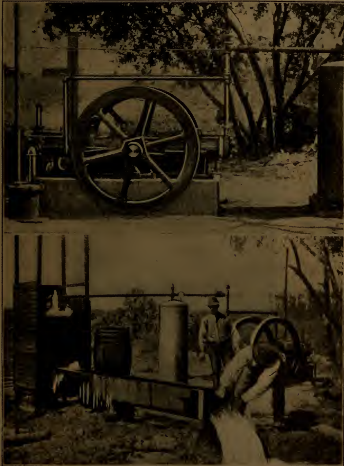
FIG. 53.—GASOLINE AIR COMPRESSING PLANT FOR PUMPING.
