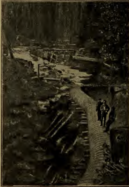
FIG. 79.—PIPE-LINE AIR COMPRESSOR PLANT AT AINSWORTH.
