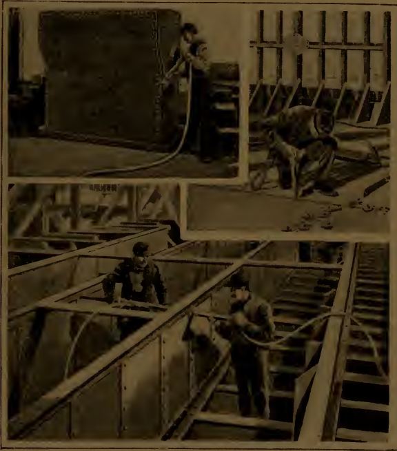
FIG. 481—CHIPPING, CAULKING AND RIVETING WITH PNEUMATIC TOOLS.
