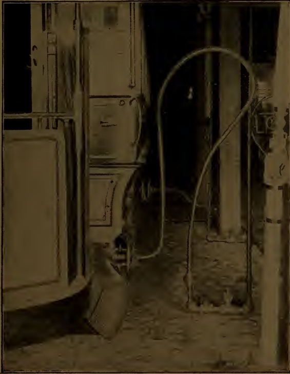
FIG. 155—CHARGING APPARATUS FOR AIR AND STEAM. THE STEAM BEING USED FOR RE-HEATING PURPOSES.
