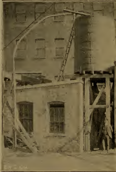
FIG. 224.—RAISING WATER BY THE POHLE AIR LIFT AT H. LANG CO.'S FACTORY, NEWARK, N. J.
