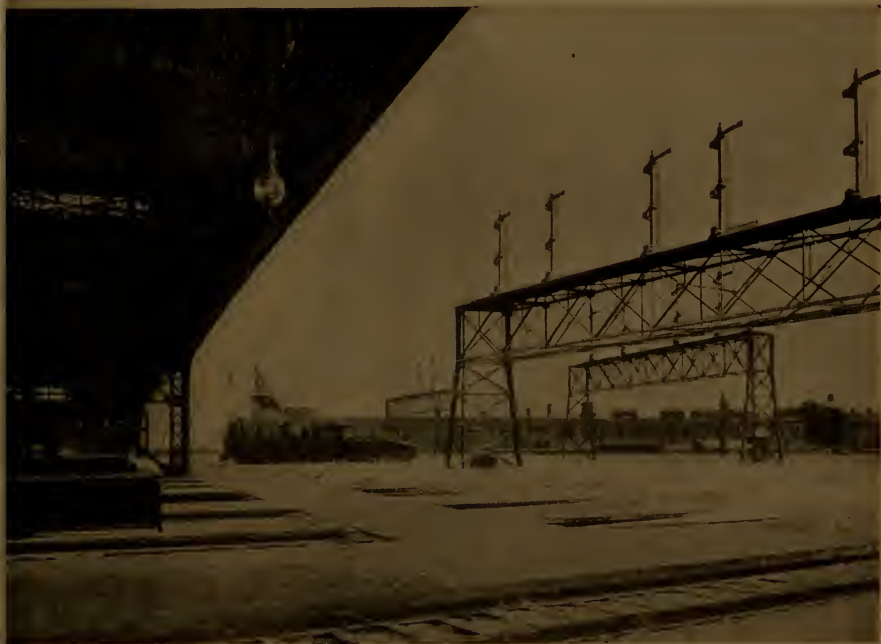
FIG. 413—BOSTON SOUTHERN STATION—WESTINGHOUSE INTERLOCKING SYSTEM DURING FEBRUARY (1899) STORM.
