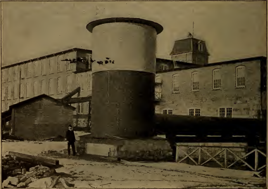
FIG. 46.—THE TAYLOR HYDRAULIC AIR COMPRESSOR.
