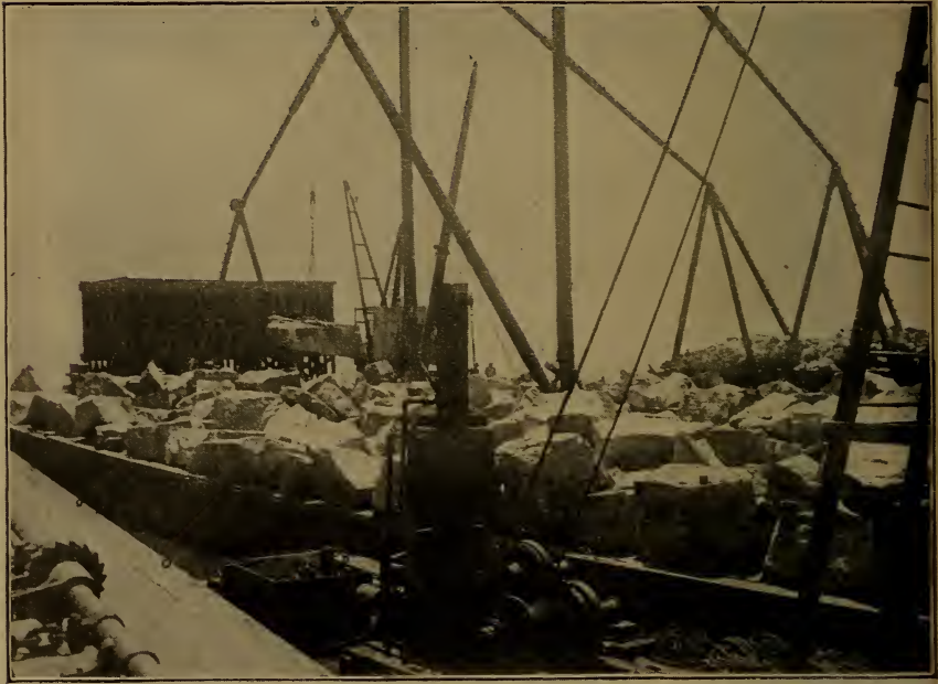
FIG. 318.—COAL-BIN 600 TONS CAPACITY, AND FLAT DECK BARGE 1,500 TONS CAPACITY.
