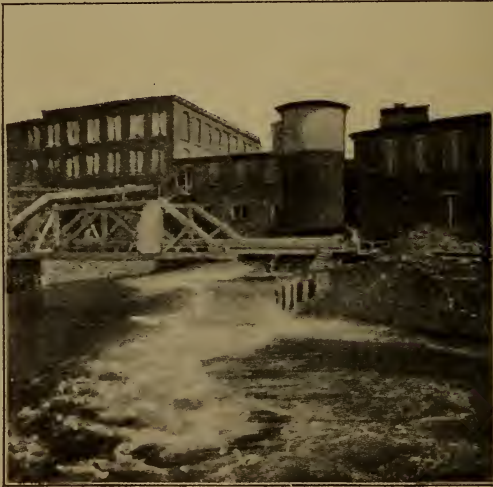
FIG. 35.—COMPRESSOR HEAD TANK AND WEIR.
