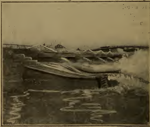
FIG. 34.—THE MAGOG DAM AT HIGH WATER.
