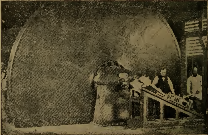
FIG. 184—PNEUMATIC DISPATCH EXPERIMENTAL WORKS AT BATTERSEA, SHOWING PNEUMATIC DISC AND ENGINE.
