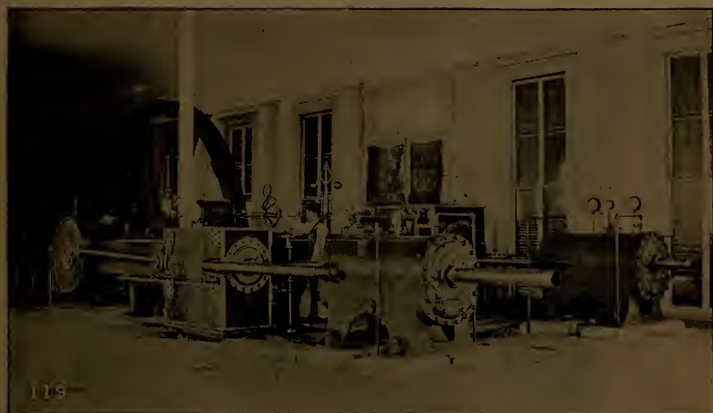
FIG. 321.—THE POWER PLANT—JEROME PARK, N. Y.
