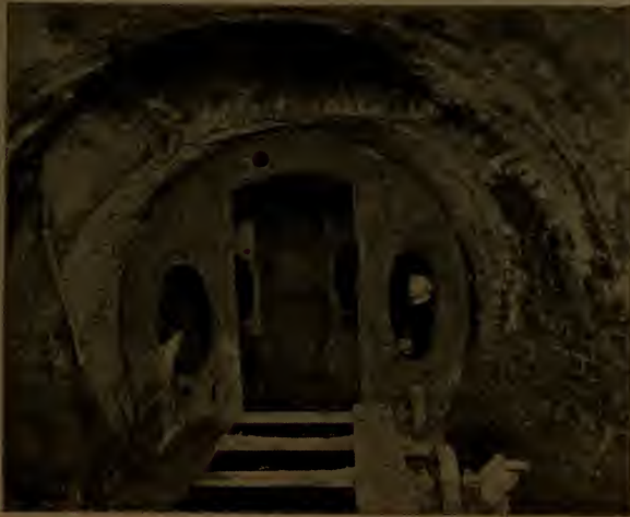
FIG. 180—PNEUMATIC CAR IN THE BROADWAY TUNNEL.
