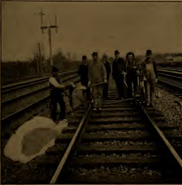
FIG. 441—SURFACING RAILROAD TRACK BY MEANS OF COMPRESSED AIR.
