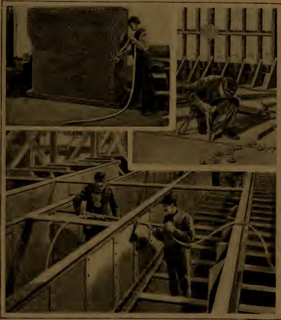
FIG. 481—CHIPPING, CAULKING AND RIVETING WITH PNEUMATIC TOOLS.
