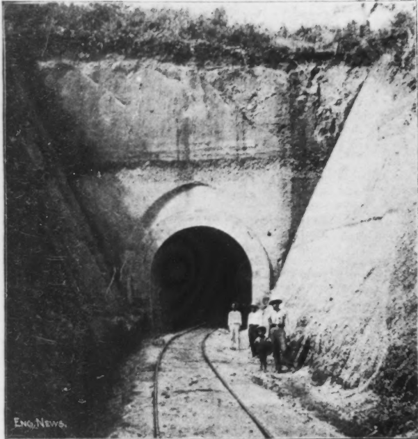
PORTAL OF TUNNEL BETWEEN MASAYA AND CATARINA.
