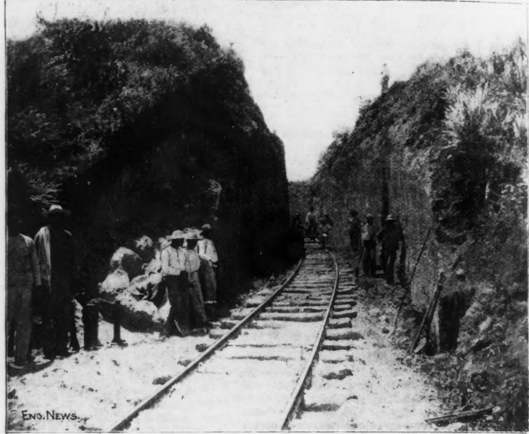
DEEP CUT NEAR TUNNEL, MASAYA-DIRIAMBIA BRANCH.
