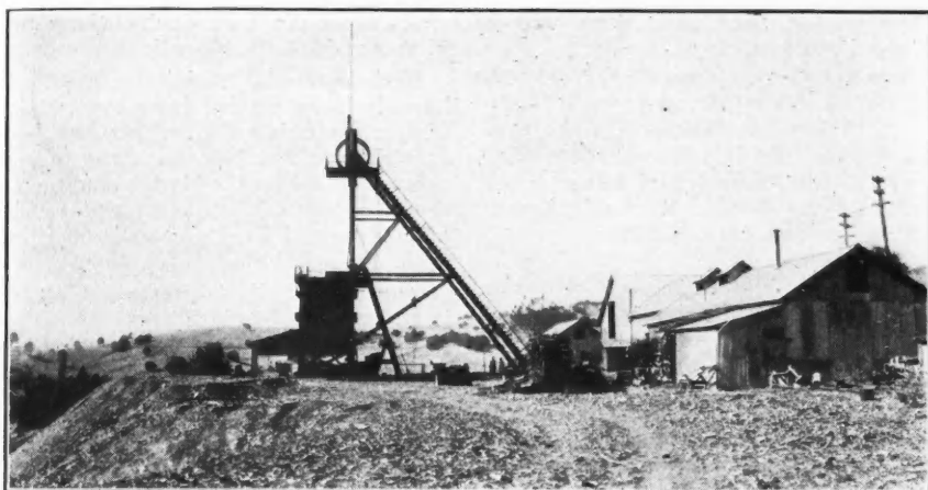
SURFACE WORKINGS AND HEADFRAME, OLD EUREKA MINING CO., SUTTER CREEK, CAL.
