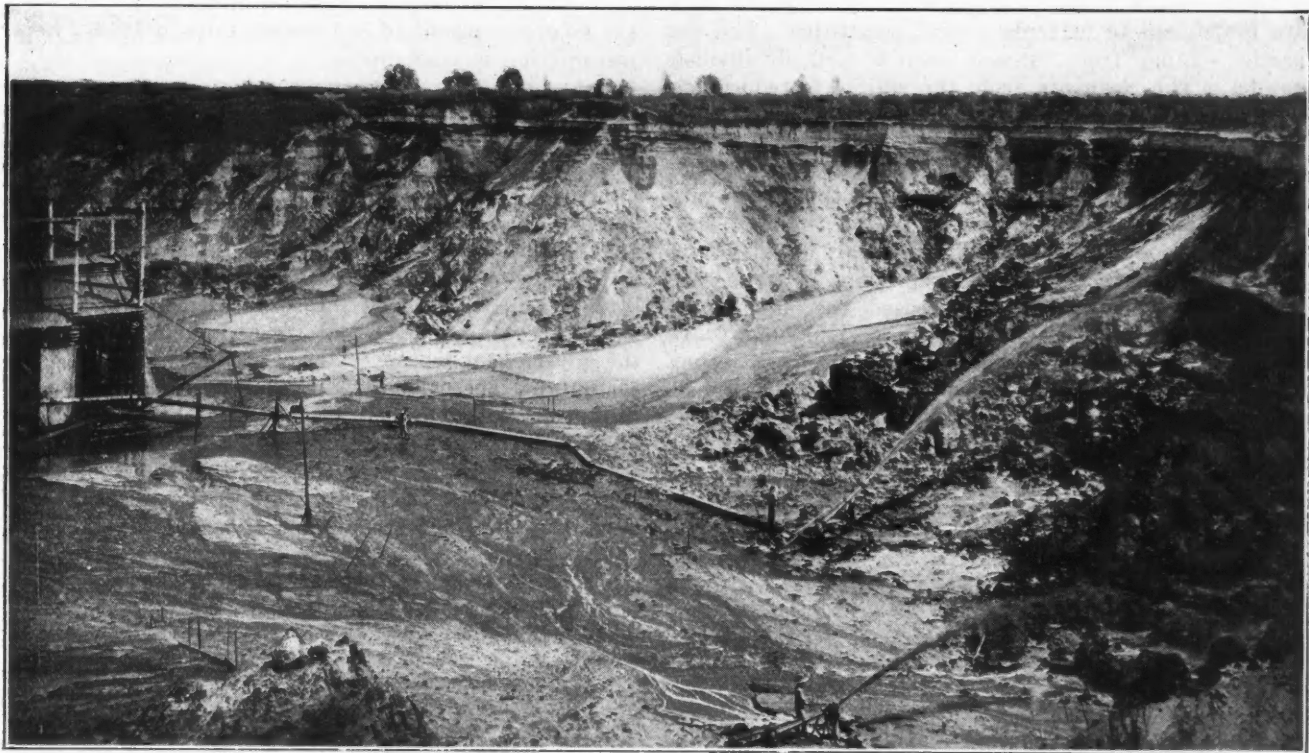
HYDRAULIC MINING ON BILLITON ISLAND, DUTCH EAST INDIES
