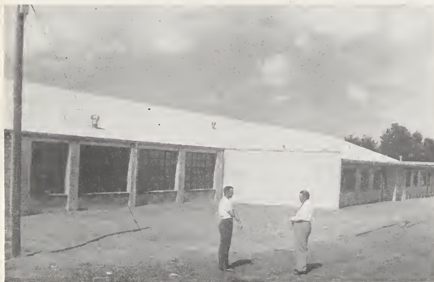
This modern $150,000 industrial building was constructed by the Franklin County Industrial Foundation to attract new industry in the area. L. D. Lowry, Jr. (left) foundation chairman, and Mt. Vernon Mayor Charles Teague check the building and layout.
