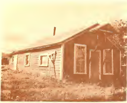
Figure 37. While appearing to be a frame structure, this building is made of log with drop siding. (Scott)
