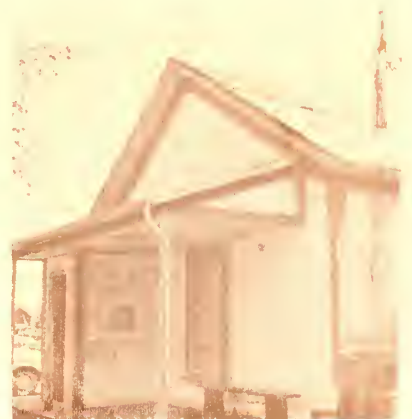
Figure 40. A frame house often has a shed roof porch with an enclosed winter entrance. (Scott)
