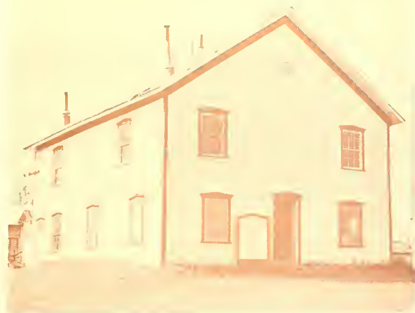
Figure 45. Today the courthouse stands without its porch and the building is used as the Eagle Public Library, a temporary jail and a museum. Plans call for its restoration in 1976. See Figure 13 for comparison. (Scott)
