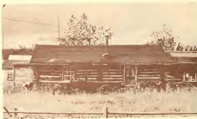
Figure 34. Log houses often had one or more rear additions. Side facades and additions had either double-hung sash or casement windows. (Scott)
