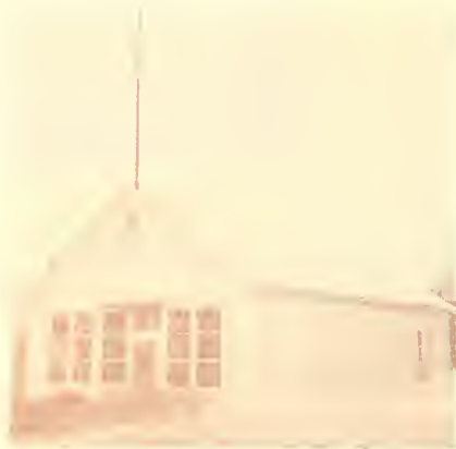
Figures 43 a and b. Large panes of glass should not be used in new buildings on B Street. The total area of glass should be divided by vertical and horizontal muntins similar to those in the Taylor building (left), or the NC Company store (right). (Scott)
