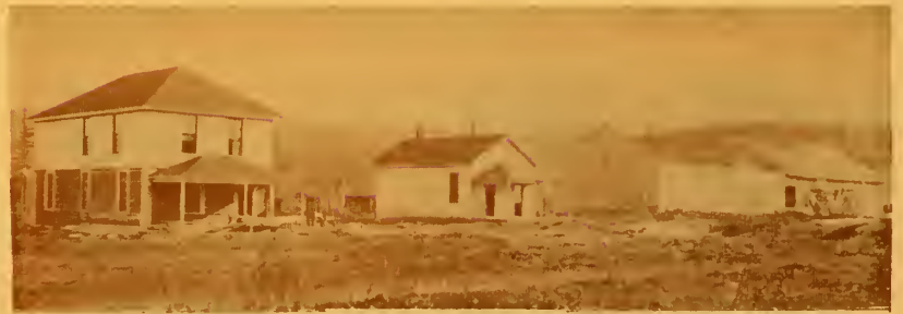
Figure 8. Post administration building and guardhouse with commissary under construction, 1901. Exterior was sheathed in corrugated iron after carpentry work was completed. (National Archives)
