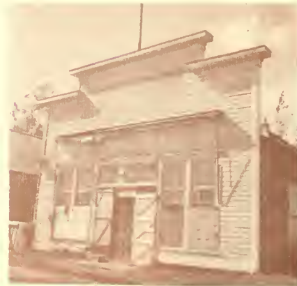
Figures 43 a and b. Large panes of glass should not be used in new buildings on B Street. The total area of glass should be divided by vertical and horizontal muntins similar to those in the Taylor building (left), or the NC Company store (right). (Scott)
