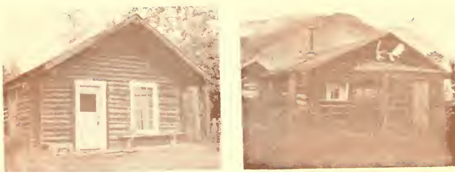
Figures 33 a and b. Windows in the gable walls of Eagle's log cabins are either double-hung sash with six-lights-over-six, as shown in cabin with the overhang (a), or three-lights-over-three casement windows, as shown in cabin without the overhang (b). (Scott)
