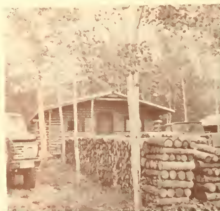
Figure 36. This new log cabin relates well to the traditional design elements of Eagle's older log houses. (Scott)
