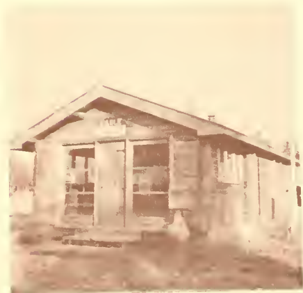
Figure 35. The new Eagle Post Office, built of tongue-and-groove logs, relates well to Eagle's older log buildings. (Scott)
