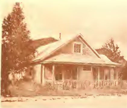
Figure 39. Eagle's frame houses also have gable roofs and face the front property line. The entrance is located in a gable wall and is usually flanked by one or two windows, commonly double-hung sash. Most of the houses are one and one-half stories high. (Volz)
