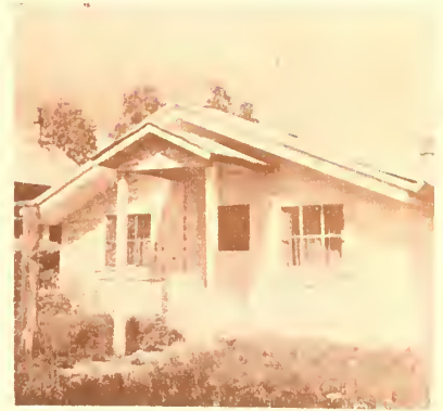
Figure 38. The Amundsen cabin is actually built of logs that were later covered with siding. Its basic form is more that of a log structure than a frame structure. (Scott)
