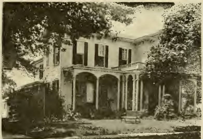
RESIDENCE OF GORTON D. JERAULD, Corner South and 6th Streets.
