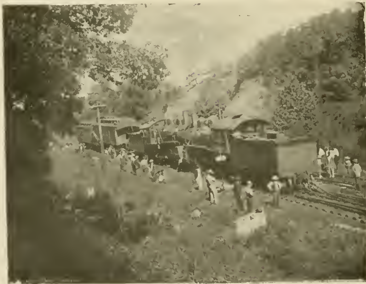
Wreck on Vandalia Line night of June 29, 1897, near the paper mill. Above picture shows the telescoped engines, the demolished coaches having been detached and dragged away.
