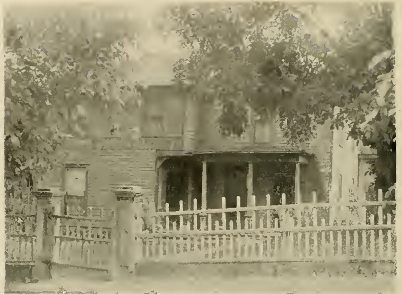
RESIDENCE OF M. J. HARDING, South Eighth Street.
