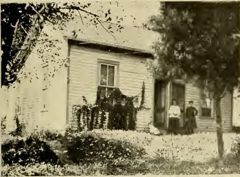
RESIDENCE OF E. C. GAINES. West Gallatin Street.
