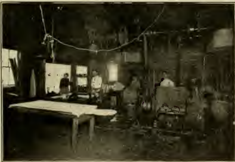
INTERIOR OF THE VANDALIA STEAM LAUNDRY. E. J. Dietz, Proprietor.
