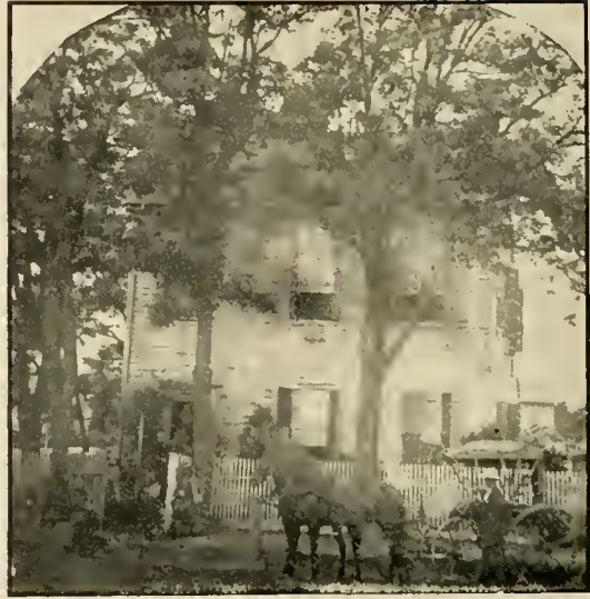
RESIDENCE OF HON P. FIELD.
