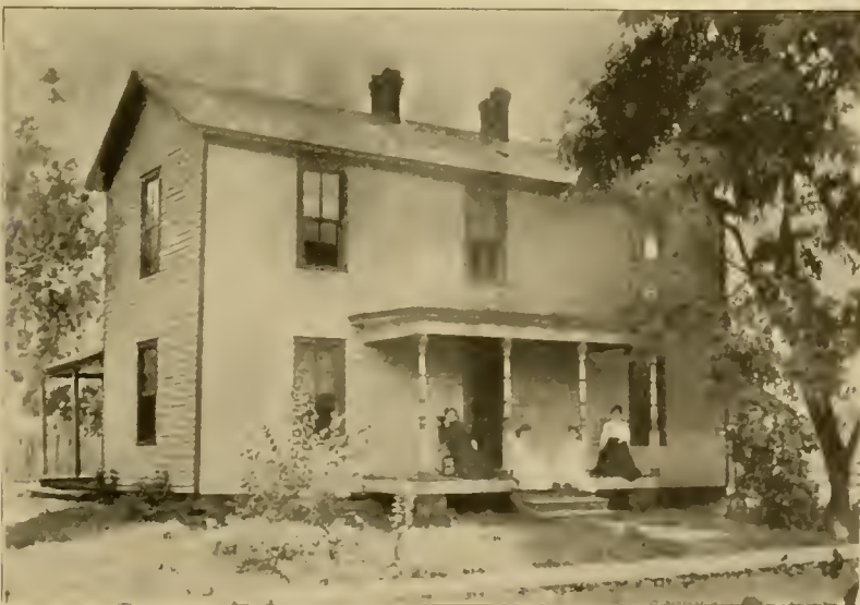
RESIDENCE OF J. H. BROWNING. West South Street.
