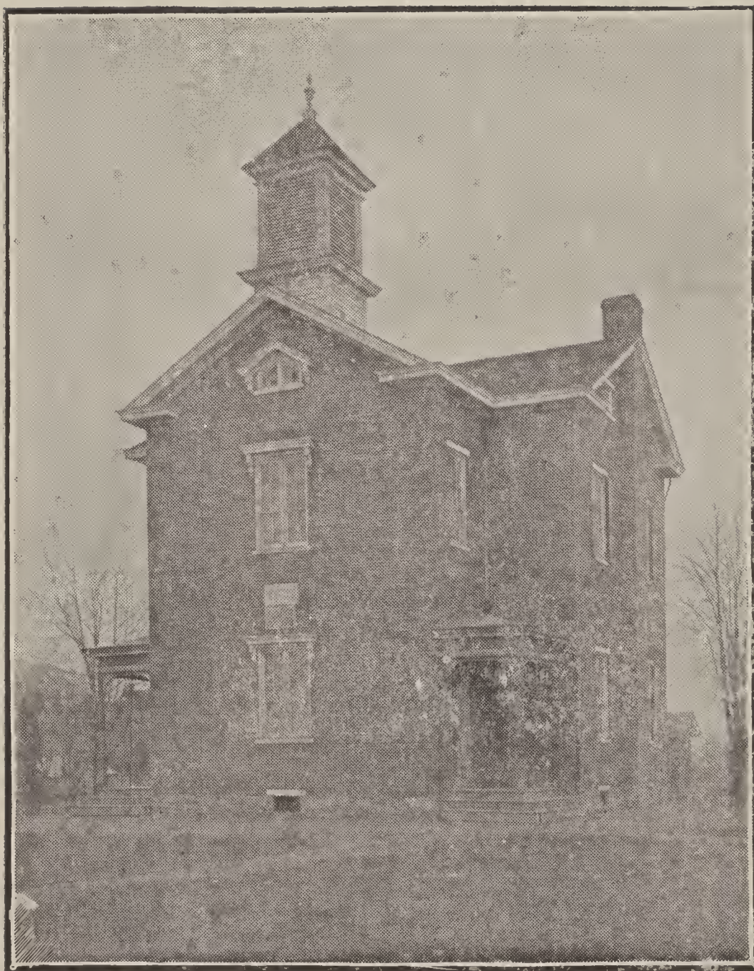
RIVERSIDE SCHOOL BUILDING.
