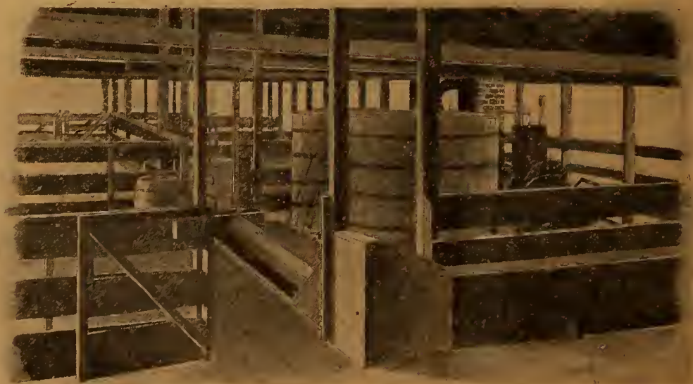
Figure 35. View of the Dipping Plant at the Stock Yards, South Omaha, Neb.
