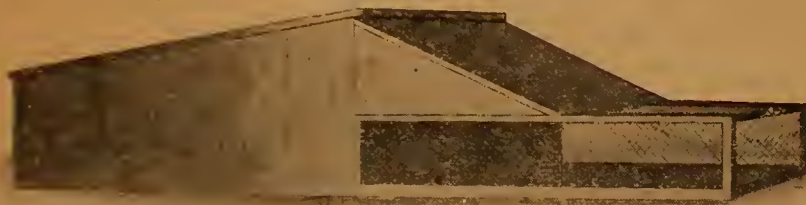
Figure 21. Chicken Coop with Enclosed and Partly Covered Run.
