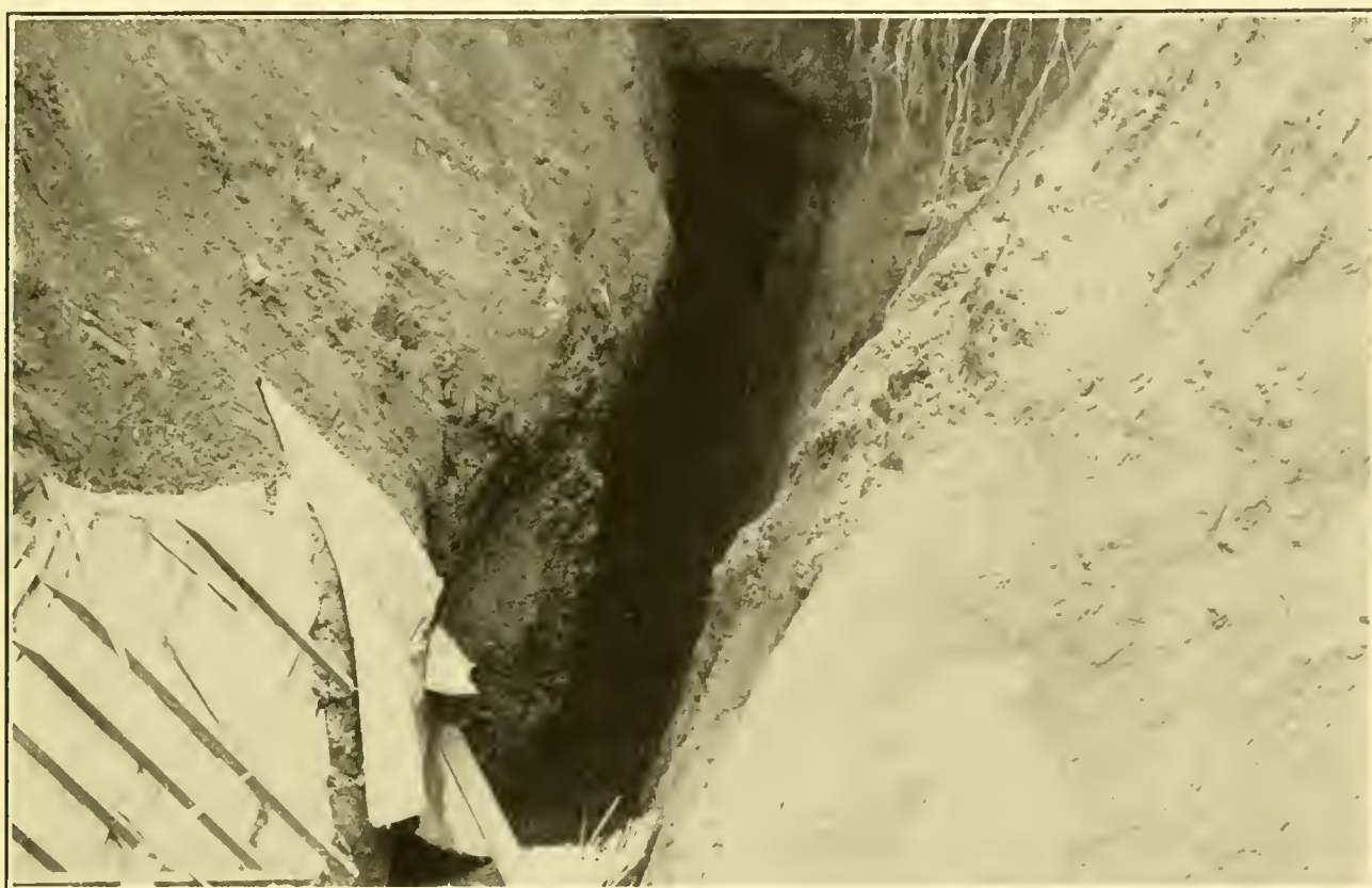
View showing the crevice opening into the limestone cavern under the Todd house.
