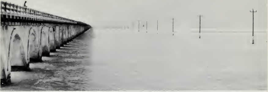
Poles set in ocean are a common feature of Florida Keys Electric.
