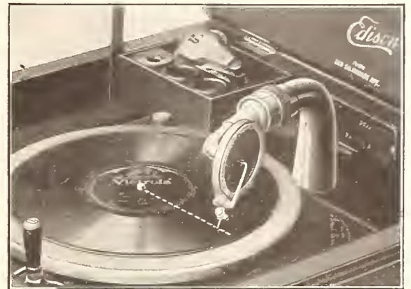
SHOWING POSITION FOR PLAYING VICTOR OR OTHER LATERAL CUT RECORDS
