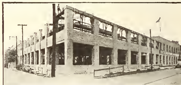
New Buescher Building Being Constructed
