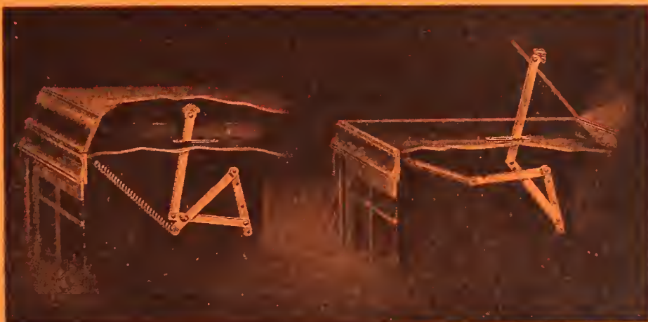
The Reproducer turns on its axis—the needle remaining on exactly the same center and at the same correct angle in both positions
