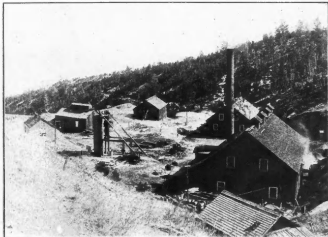
SURFACE PLANT AT THE BOSTON & ALTA COPPER COMPANY, CORBIN, MONT.
