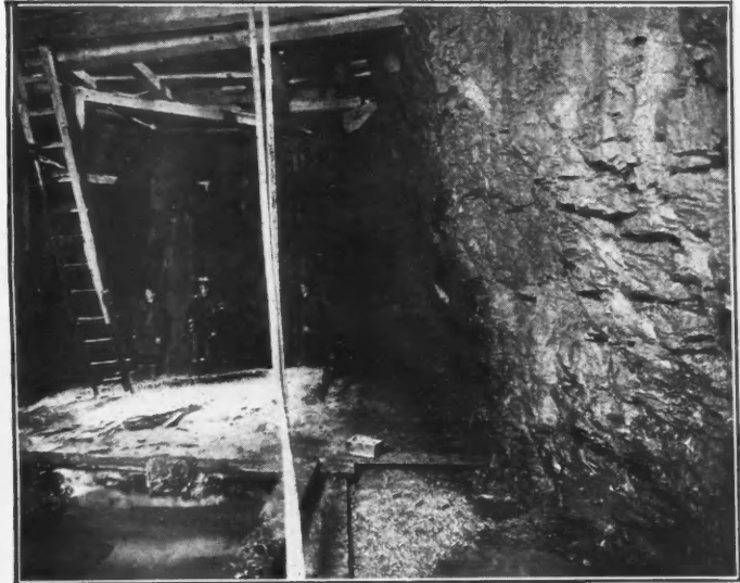
FIG. 7. EXCAVATION IN ROCK BEFORE UNDERPINNING, SHOWING CHANNELING UNDER CAISSON
