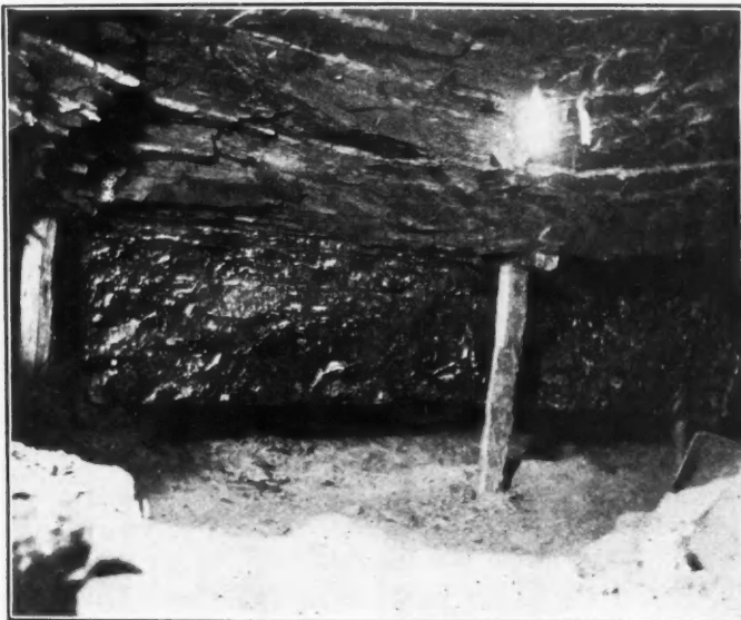
SHOWING THE LONGWALL FACE UNDERCUT AND READY TO BE WEDGED DOWN
