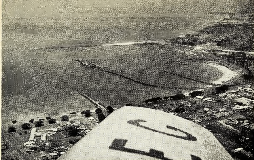
Portland Bay during early stages of construction of new harbour installations, Ocean Pier at centre.
