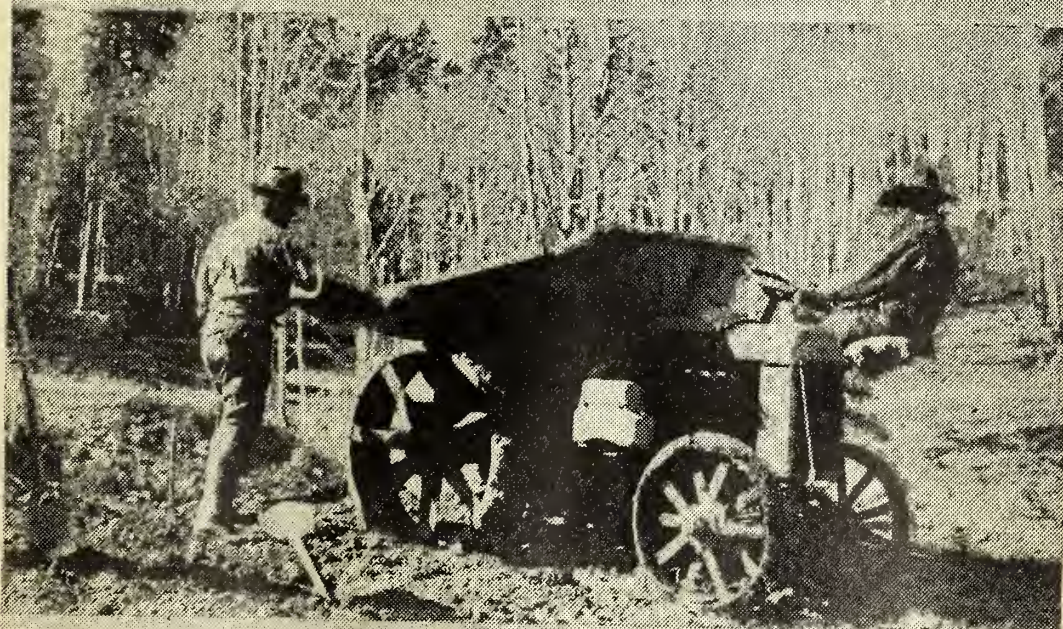
Figure 1. - (Top) The iron mules, because they are low and small, were loaded easily without being turned around at the gasoline shovel.
