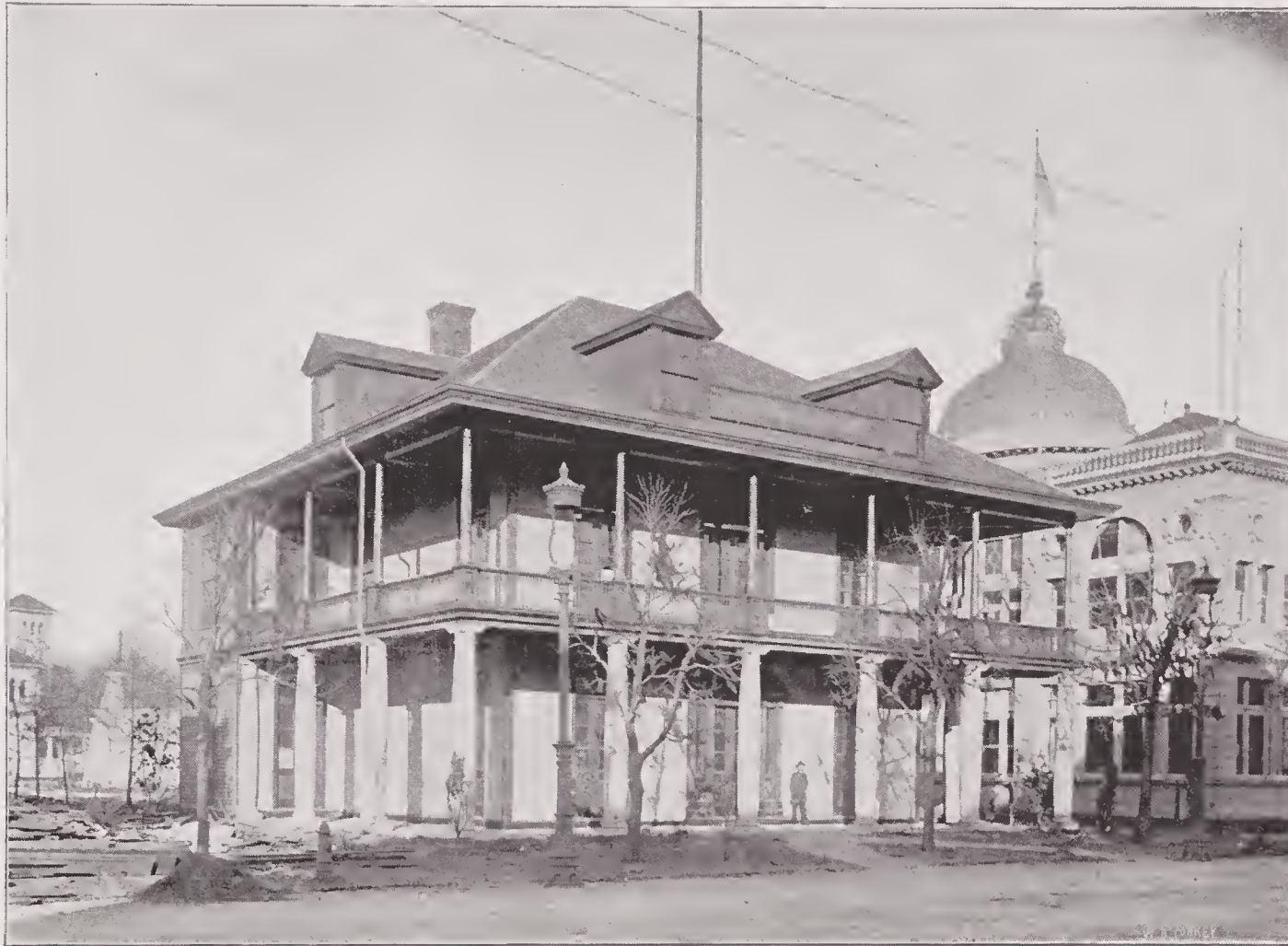
The Louisiana Building was in imitation of the old-fashioned Creole houses of the state; was two stories in height, with a piazza to each story, and was finished in native woods. Upon the second floor was a large exhibition room containing valuable and curious relics. Here Creole women showed the Acadian manner of weaving.
