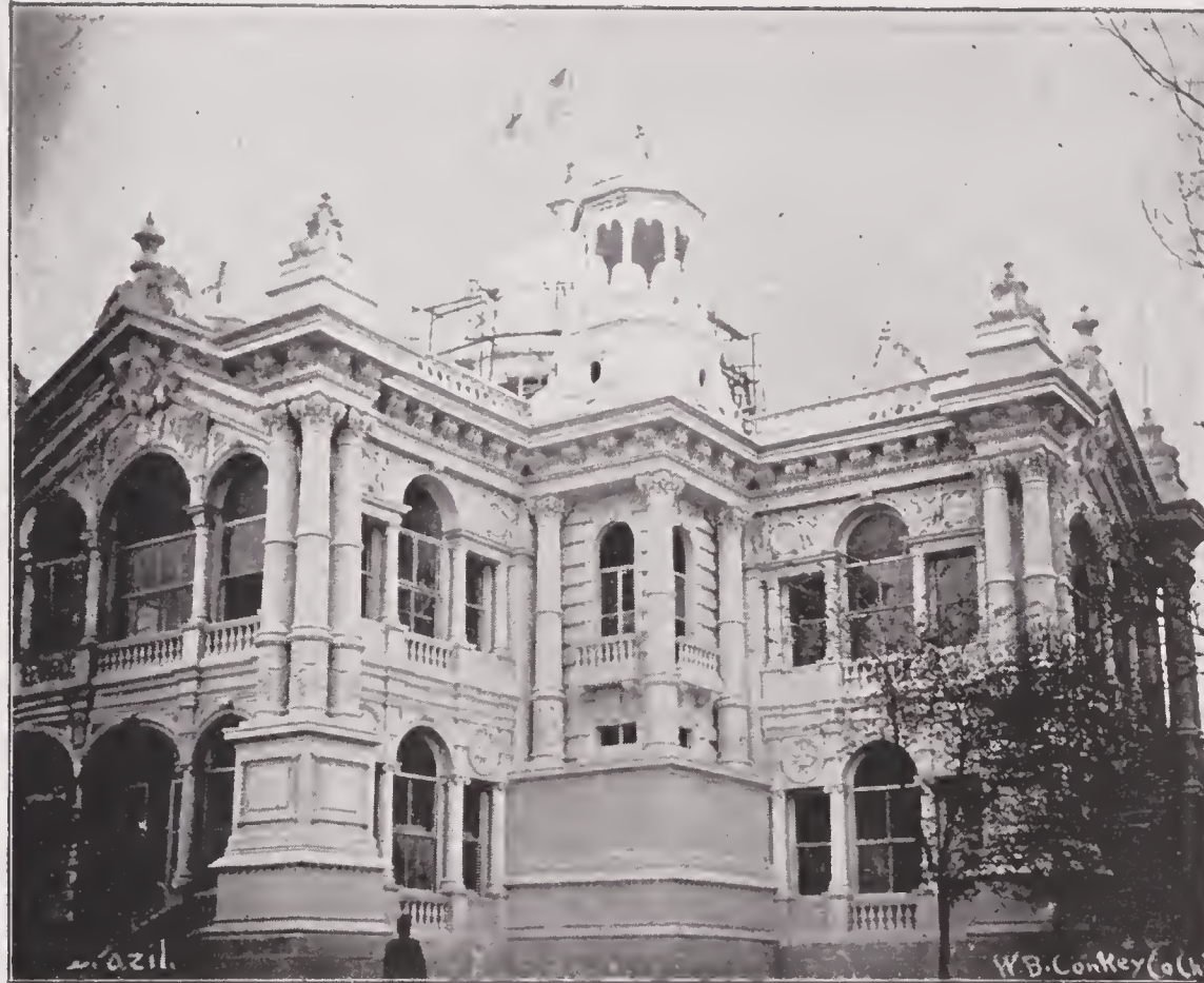
The Brazilian Building was one of the finest government structures on the grounds, occupying an area one hundred and fifty feet square, and standing in the form of a Greek cross. It was of two stories surmounted by a handsome dome. There were no exhibits here, but the interior was tastefully decorated to illustrate events in Brazilian history
