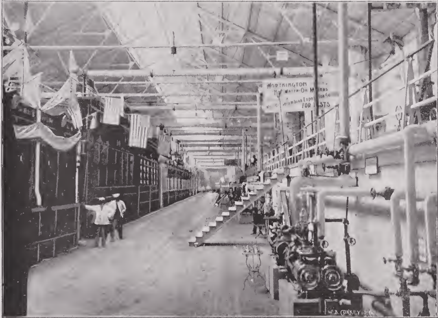
The Boiler Room of Machinery Hall was a sight worth seeing for the student of modern industrial methods. Here was arranged the greatest battery of boilers in the world, the illustration showing its enormous length. No coal was used, the fuel supplied being entirely of kerosene oil. The soul of Watts would have been delighted with the spectacle.
