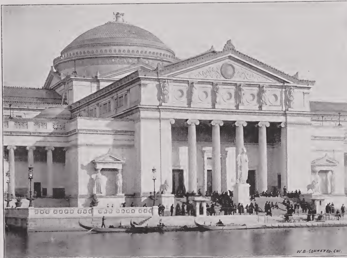
The southern entrance to the Art Palace was a favorite spot for visitors to the World's Fair, not only because here was a convenient landing place for boats, but because the view to the south was one of great extent and beauty. The illustration gives an excellent idea of some of the details of architecture of this famous edifice.
