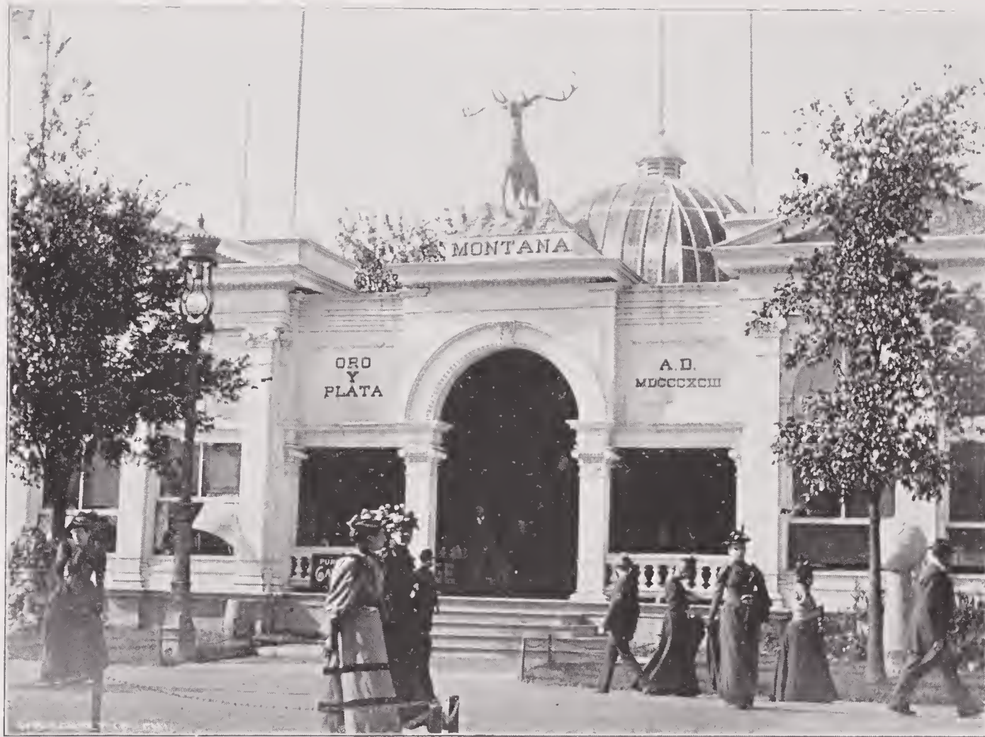
The Montana Building was of the Romanesque style of architecture and but a single story in height and costing $16,000. It was surmounted by a glass dome twenty-two feet in diameter and thirty-eight feet high. Panels in pure sheet gold were among the decorations from this mining state. The figure of a gigantic elk appeared above the entrance.
