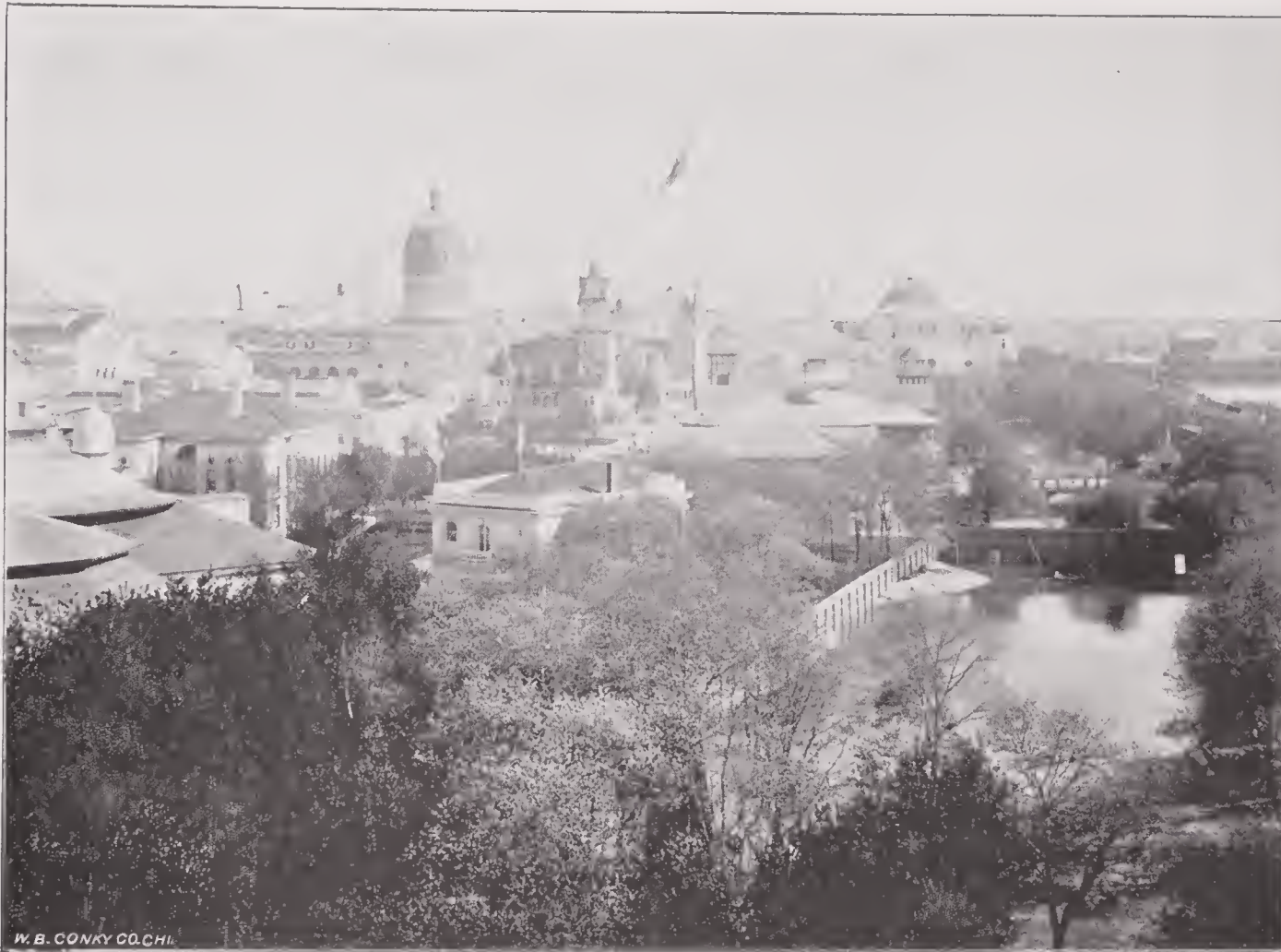
At the northwest corner of the grounds a view to the southeast was something most attractive. Close at hand to the right was the pretty isolated northwest pond, and to the left extended a panorama of state buildings with the domes of the grander structures showing above them in the remote distance.
