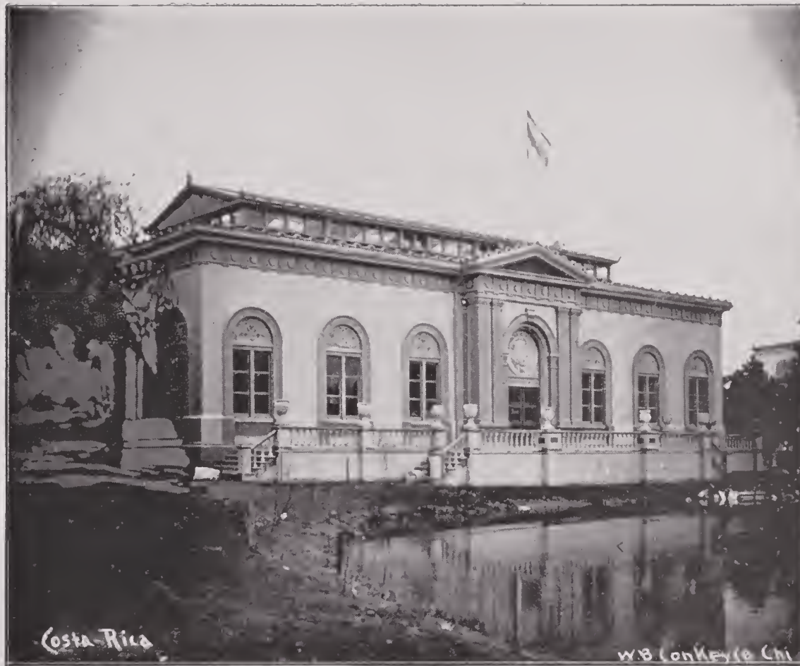
The Costa Rica Building, situated at the east end of the North Pond and facing west, showed to advantage its pure Doric style. In the construction much iron and cement were used, the whole being tastefully painted. The display made of tropical birds and plants added greatly to the attractions of the interior of the edifice.
