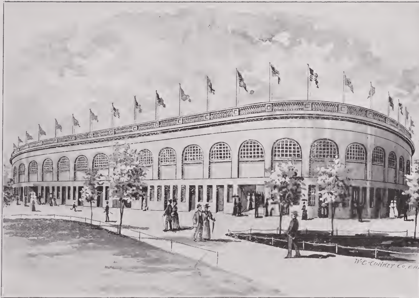
The Live Stock Pavilion, in the arena of which the parades of live stock and competitive displays were made, was an immense structure in the southern part of the grounds. The arena alone was four hundred feet in diameter, and the ascending tiers of seats about it could accommodate fifteen thousand people at one time.
