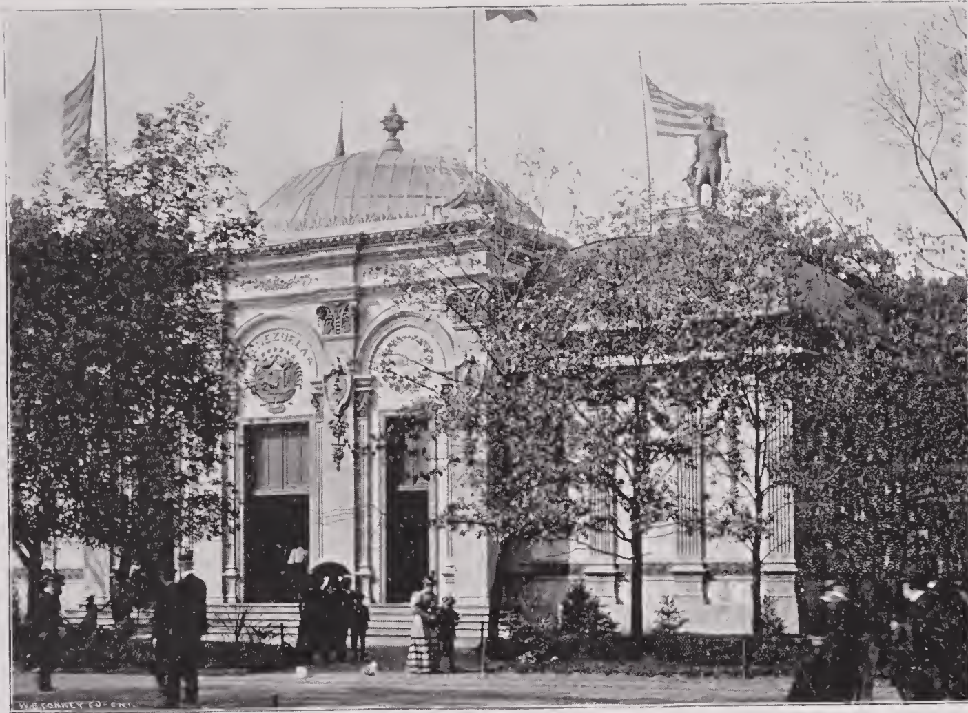
The Venezuela Building was a graceful structure of white marble, a single story in height, designed in the Greco-Roman style, and was largely the donation of public-spirited citizens of the republic. Its exhibits were most valuable, including among other relics the flag carried by Pizarro hundreds of years ago, in his conquest of Peru.
