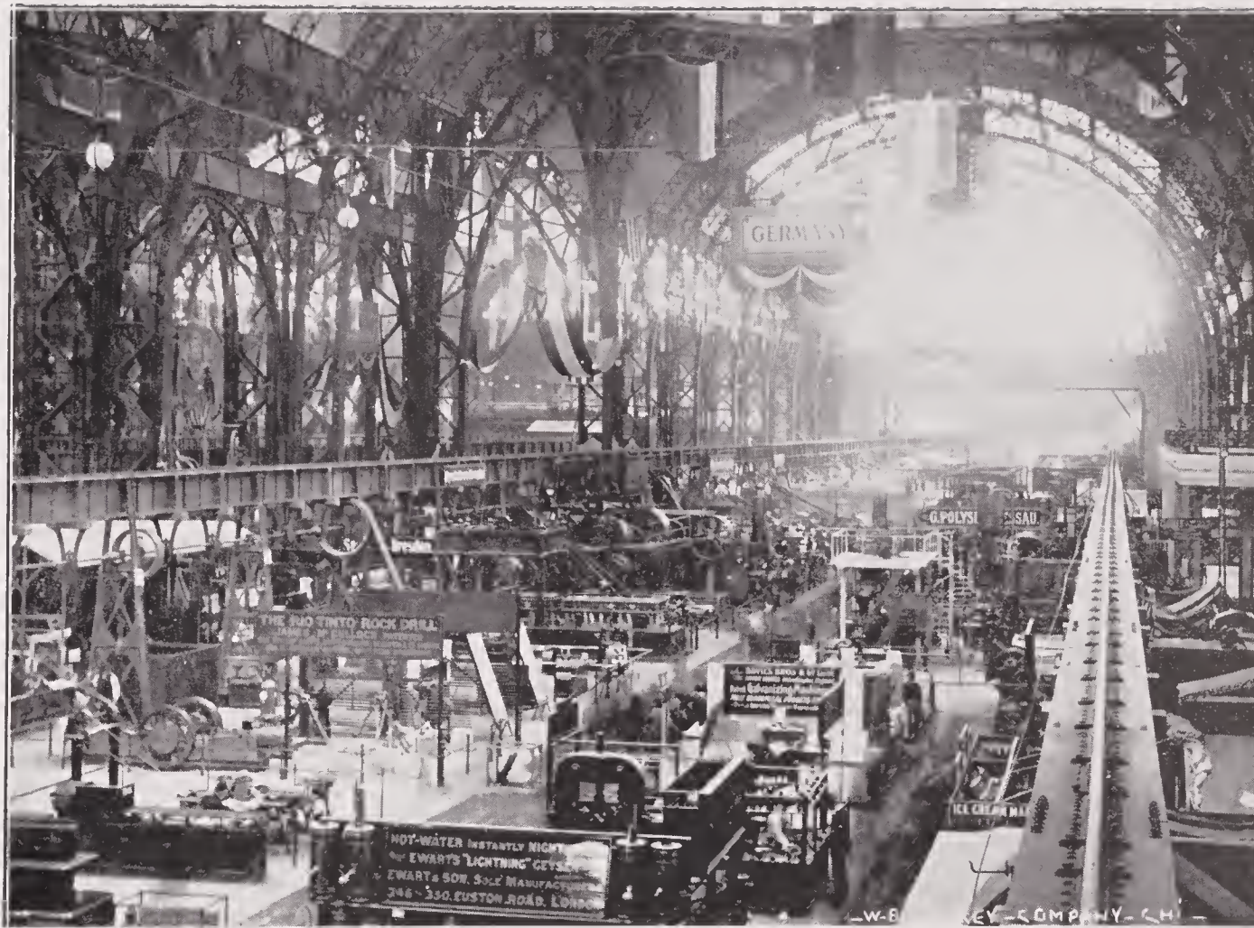
Machinery Hall was spanned by three arched trusses, and when denuded of its exhibits presented the appearance of three huge railroad train houses arranged side by side. The illustration gives a view of the nave which contained the British exhibits starting at the northeast corner, the German, New South Wales and several other foreign displays in the distance, and in the far perspective the dim outlines of the Annex.
