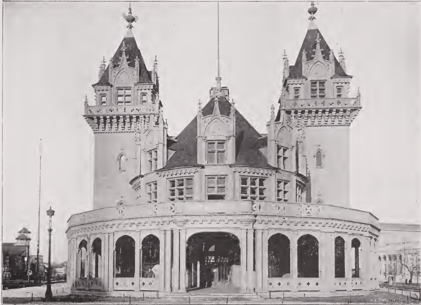
The Indiana Building was an attractive and comfortable structure built at a cost of about $65,000. It was in the French Gothic style, three stories in height, with a wide veranda and bearing two towers one hundred and fifty feet in height. It was headquarters for people from the state, making no feature of exhibits.
