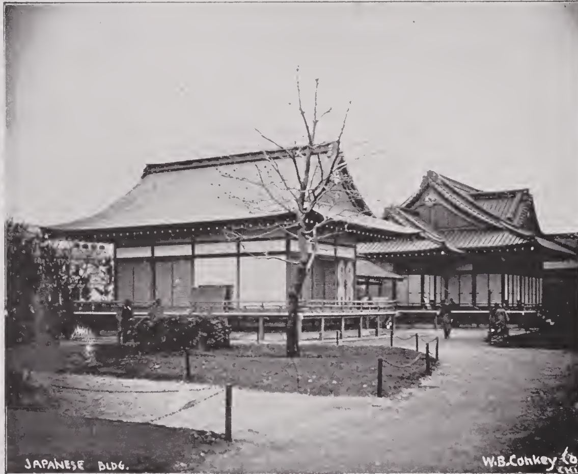
The Japanese buildings were the only structures of note on the Wooded Island and consisted of three parts connected. The style was that of an ancient Japanese temple and the buildings were illustrative in design of the methods prevailing at different periods in Japanese history. The effect of the whole was most picturesque and pleasing.
