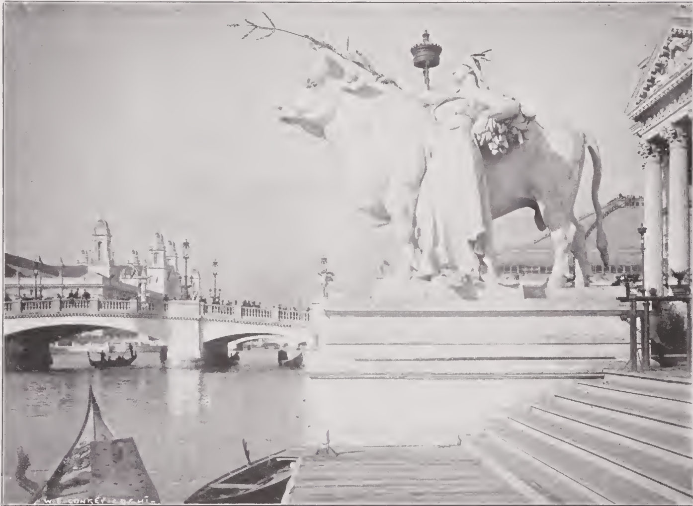
From the west front of the Agriculture Building standing beside one of the statues of Plenty, and looking northwest, the scene was most picturesque in a strictly artificial way. There was nothing of nature to the scene save the water of the canal in front, but the architectural effect was graceful in the extreme.
