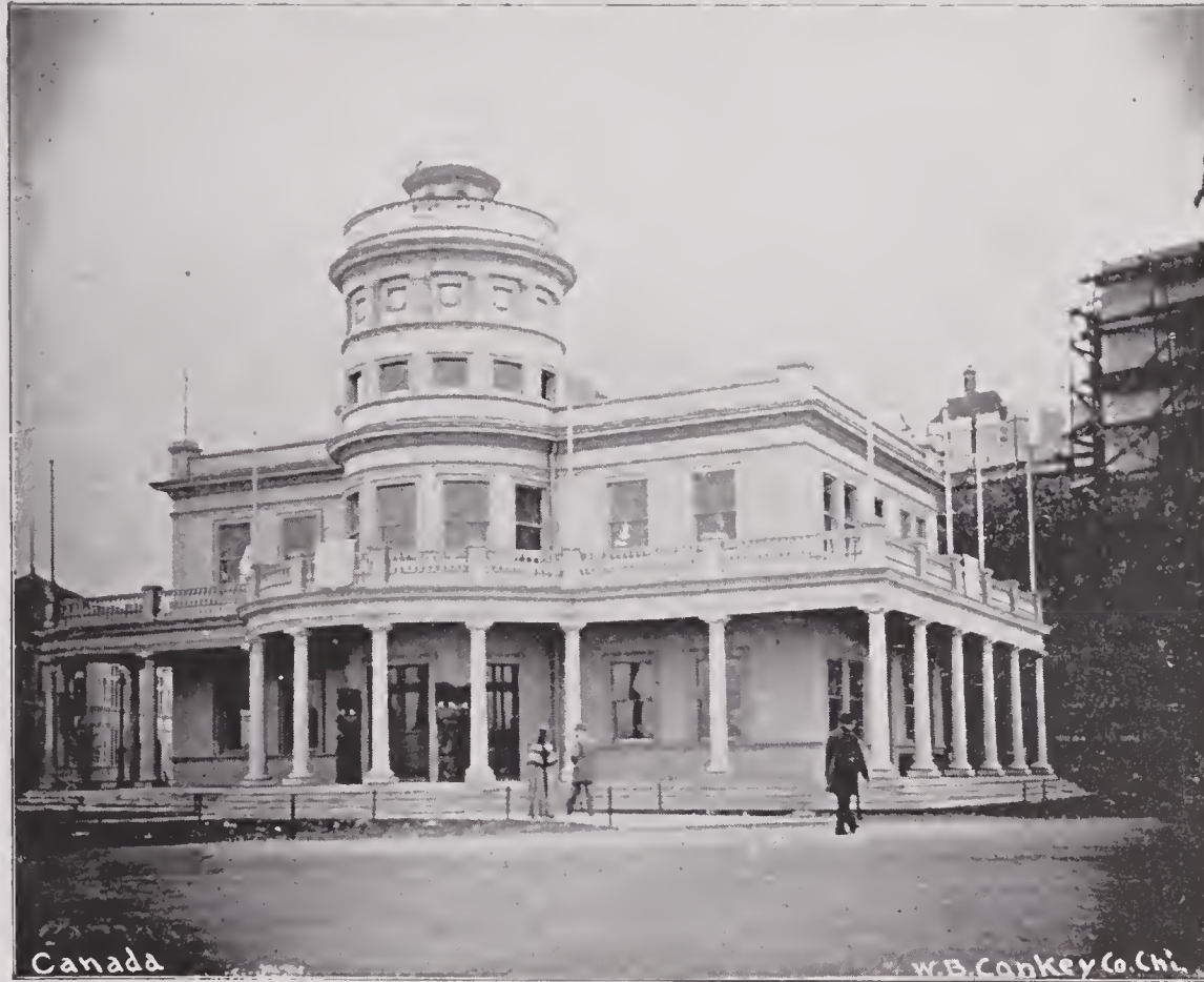
The Canadian Building, which was situated nearly opposite the British Building, on the lake front roadway, was a rather handsome wooden structure occupied by various representatives of the Dominion government. It contained a number of special exhibits from the provinces, some of them of a curious and attractive character. Its cost was $30,000.
