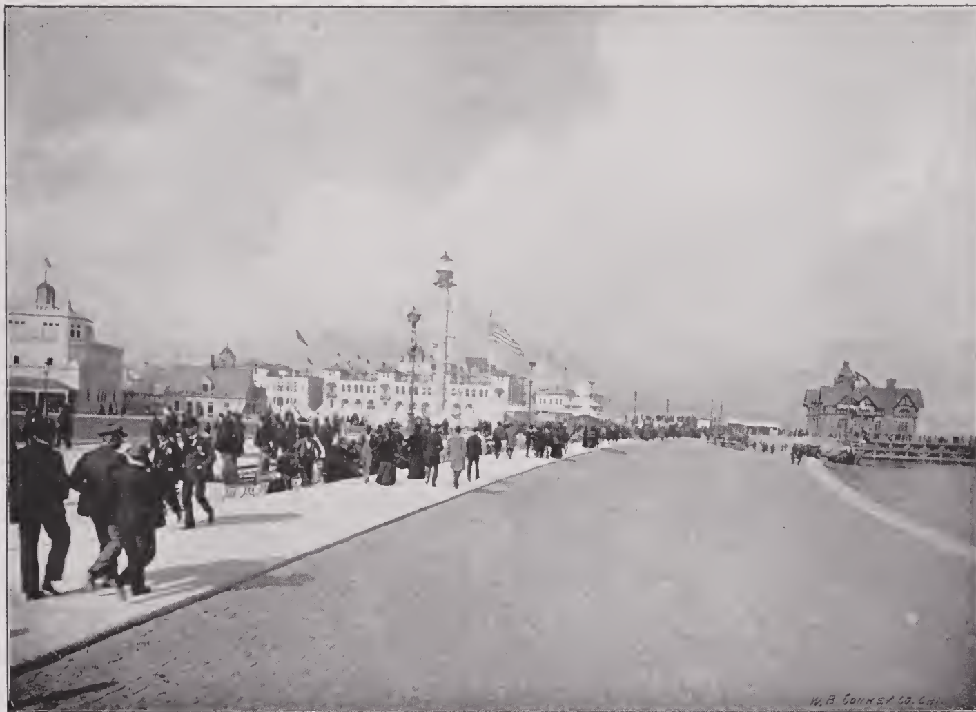
The Lake Front promenade was the great highway from the Peristyle on the south to the Naval Exhibit and the group of state and foreign buildings on the north. In the distance to the right will be noticed Great Britain's home, Victoria House, on the left the United States Weather Bureau, Life Saving Station and Observatory, and immediately in the rear the Clam Bake Building.
