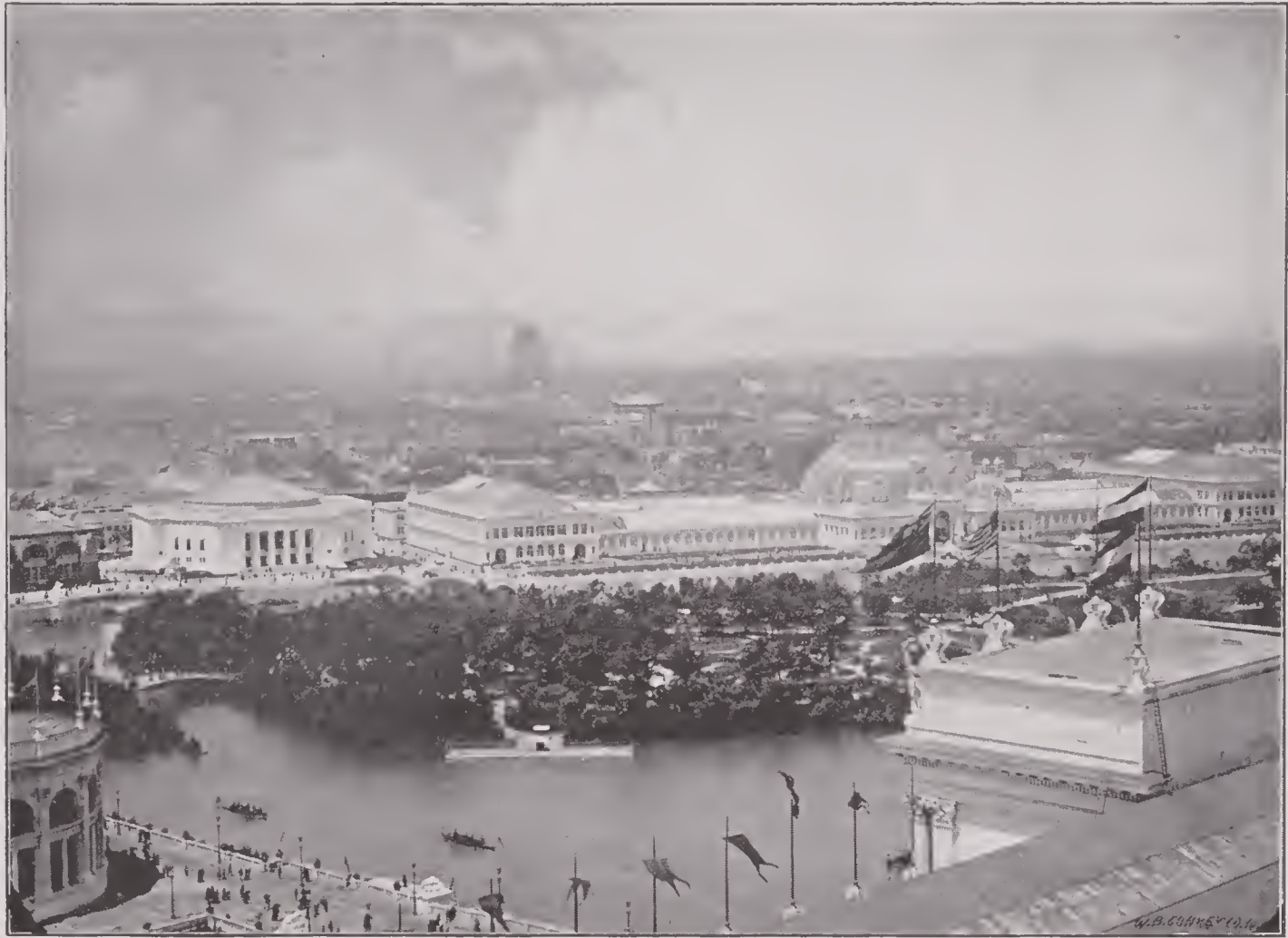
The Wooded Island, viewed from the roof of the Manufactures Building, lay beneath the eyes in such a manner that all its features could be perceived. In the view given above, the south half of the Island is particularly well defined. The object lying beside the Island in the foreground is the float, whereon performances were sometimes given.
