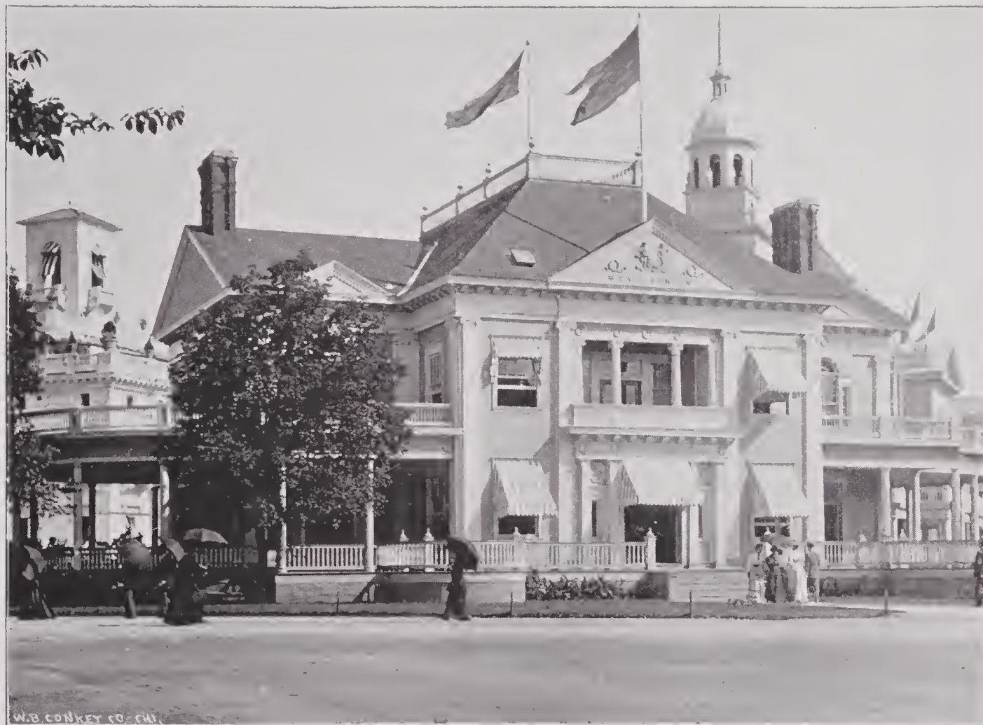
The West Virginia Building was in the Colonial style, representing a West Virginia residence, and was two stories in height, with a pitched roof. All the exposed material was produced in the state. The ceilings were of ornamental iron work, made in Wheeling. There were four large fireplaces, two on each floor. The building cost $20,000.
