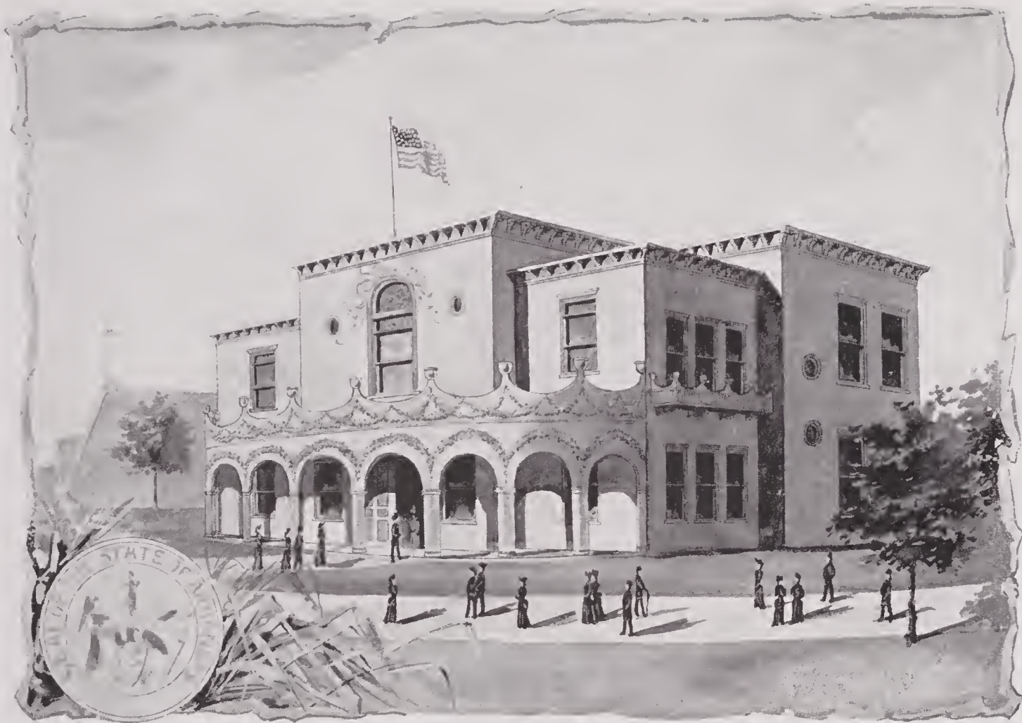
The Arkansas Building, situated near the northwest corner, was in the French Rococo style of architecture and was erected at a cost of $15,000. The exterior was in plaster and ornamental staff work, and made an excellent effect. Around the interior rotunda were six rooms for exhibits of historic interest. Some of the interior decorations were especially striking.
