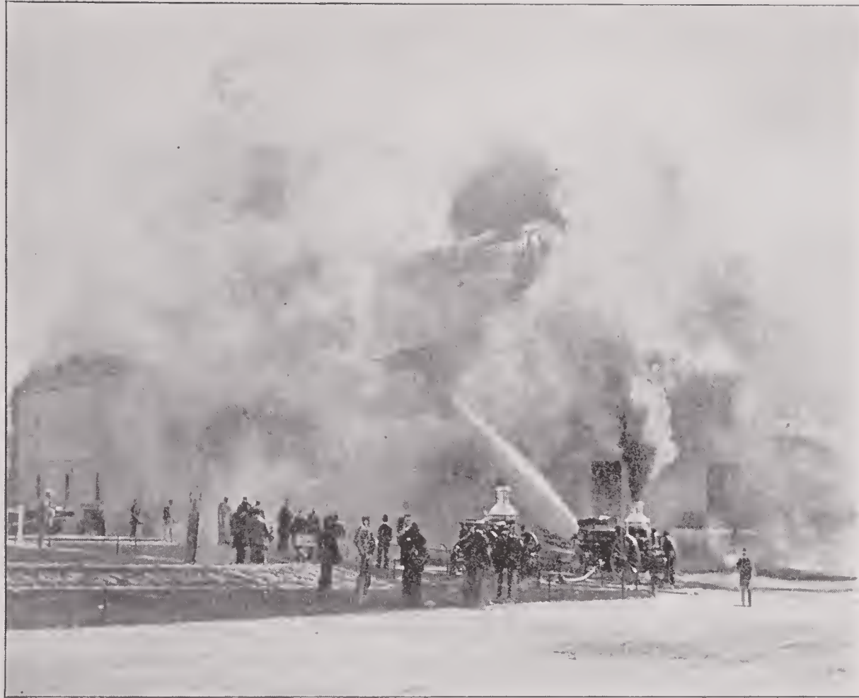
The struggle with the flames on the occasion of the Cold Storage Warehouse fire in the Fair grounds was a helpless one. Of the men cut off from escape, sixteen were lost and several others were more or less seriously injured. At least fifty thousand horrified spectators were witnesses of the appalling scene.
