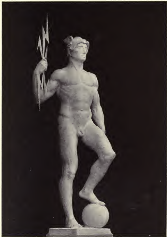
ELECTRICITY, PALACE OF MACHINERY
