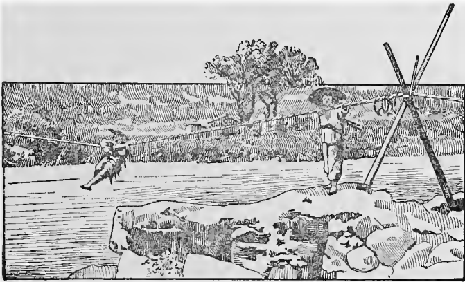
ROPE BRIDGE NEAR TA-CHIEN-LU.
