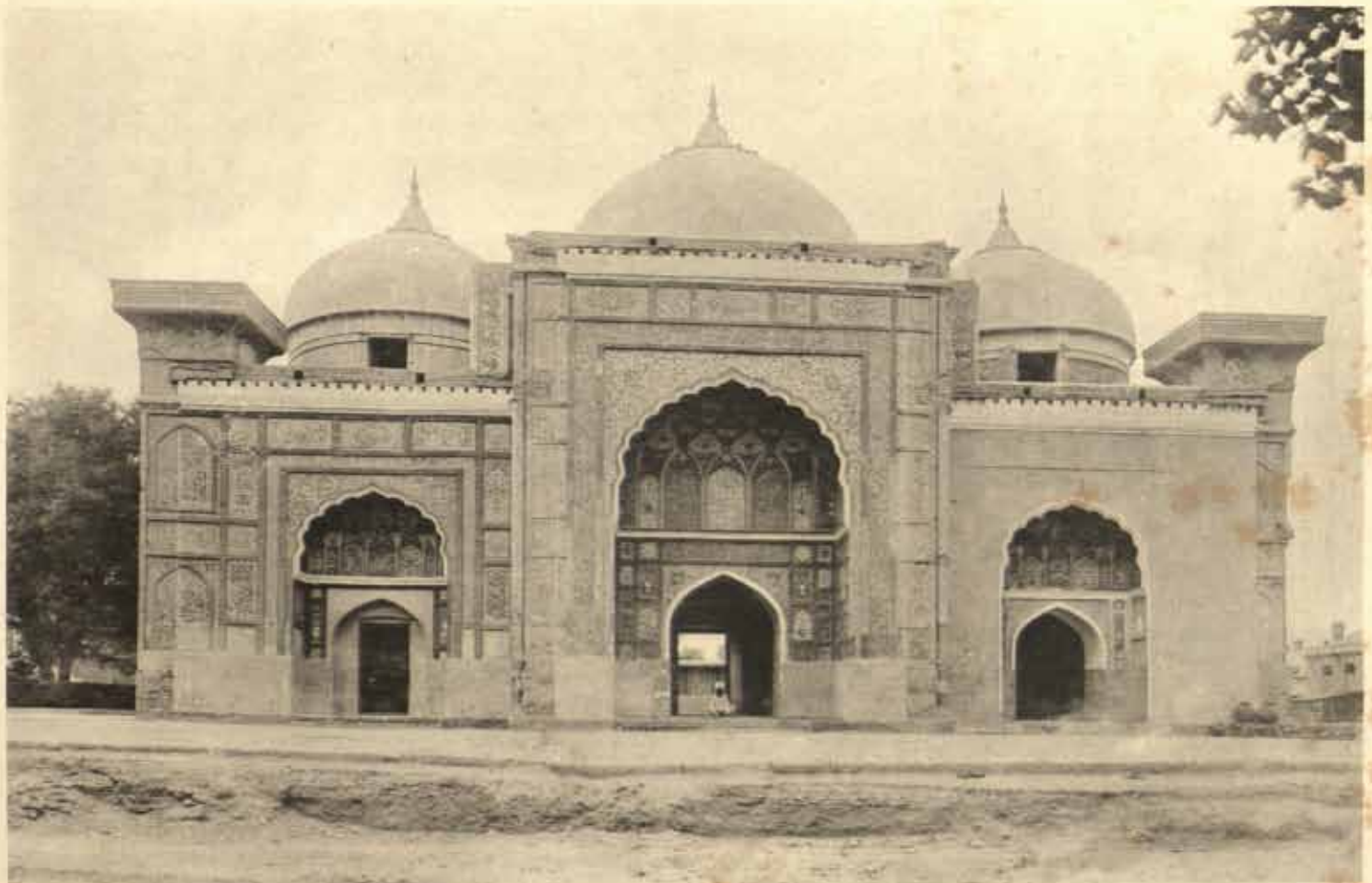
(a) SHOWING MOSQUE WHEN USED AS A RAILWAY OFFICE. (b) AFTER DEMOLITION OF MODERN ADDITIONS AND PARTIAL REPAIR.
