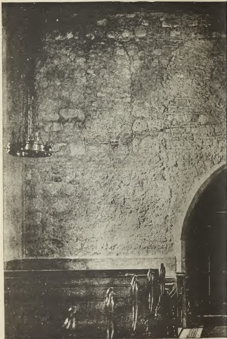
WEST WALL OF NAVE, AND ROMAN (?) WINDOWS W
