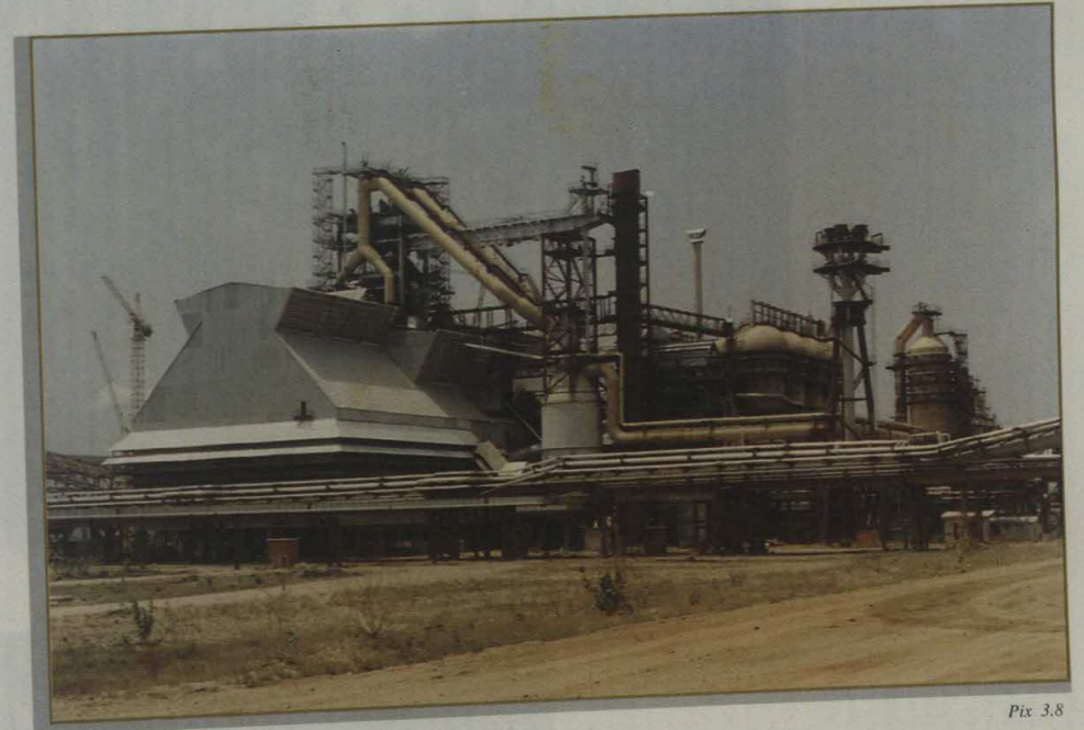
Blast Furnace capable of producing 1.3 million tonnes of liquid iron a year
