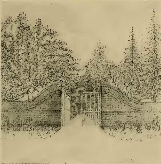
Old Southern Wall with Moulded Brick Cap
