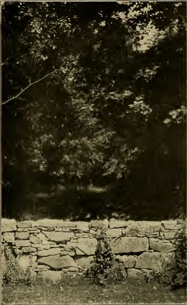
Old Stone Wall.
