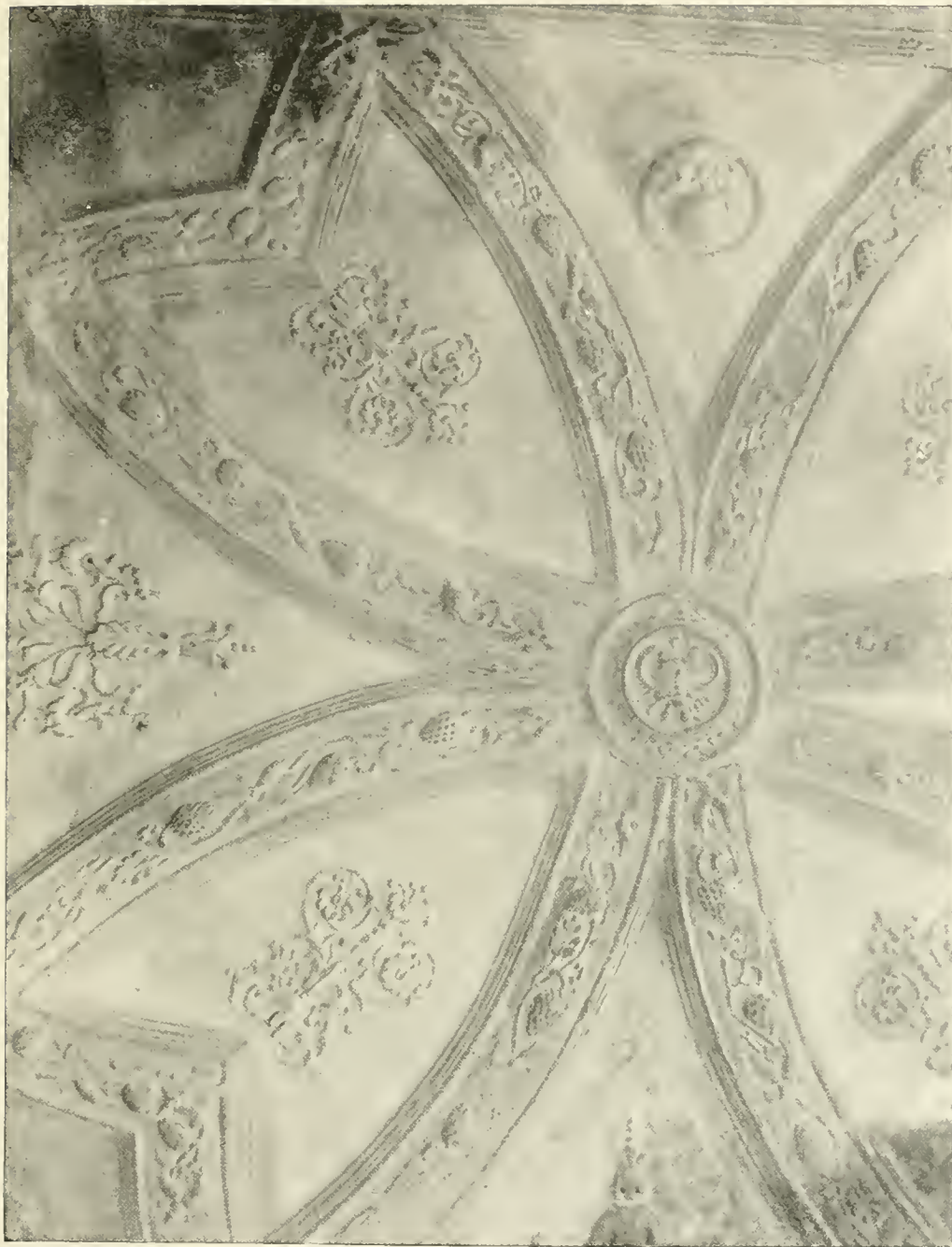
PART OF CEILING OF ROOM, FIRST FLOOR.
