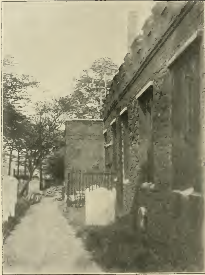
The North Aisle Wall and Old Vestry.
