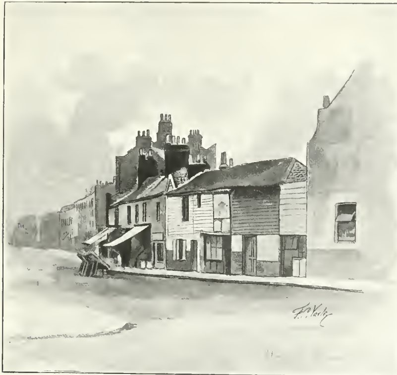
VIEW FROM NORTH-EAST
