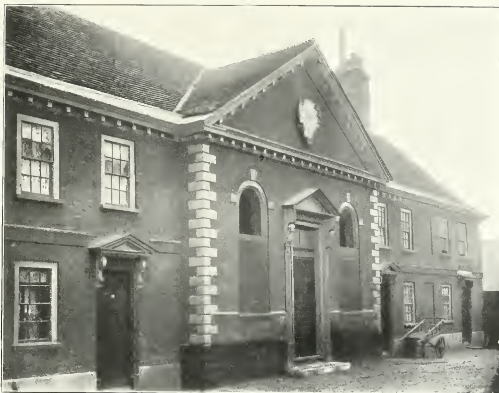
VIEW FROM NORTH-EAST.
