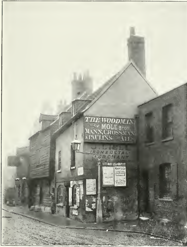
VIEW FROM NORTH-EAST.
