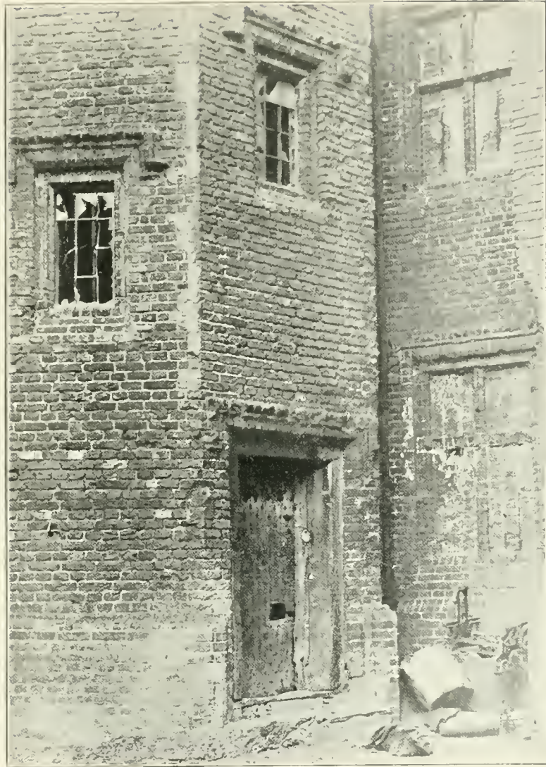
EASTBURY HOUSE, BARKING. PART OF TOWER IN COURTYARD.
