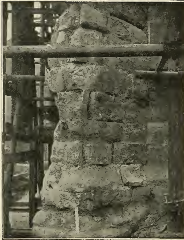
The South-West Buttress of the Tower.
