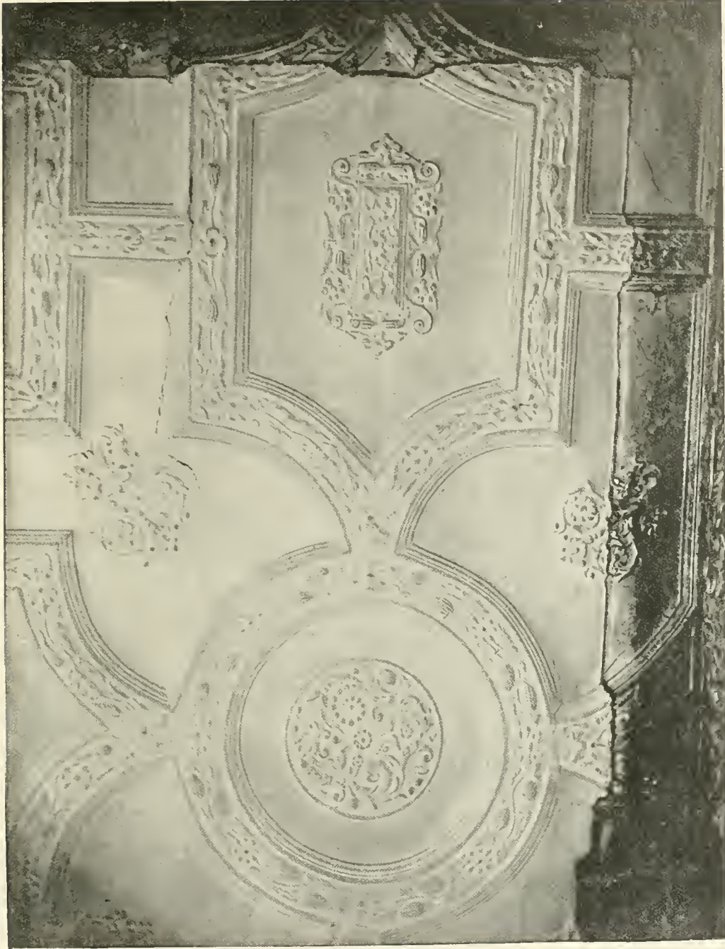
CEILING IN NORTH-WEST ROOM, GROUND FLOOR.
