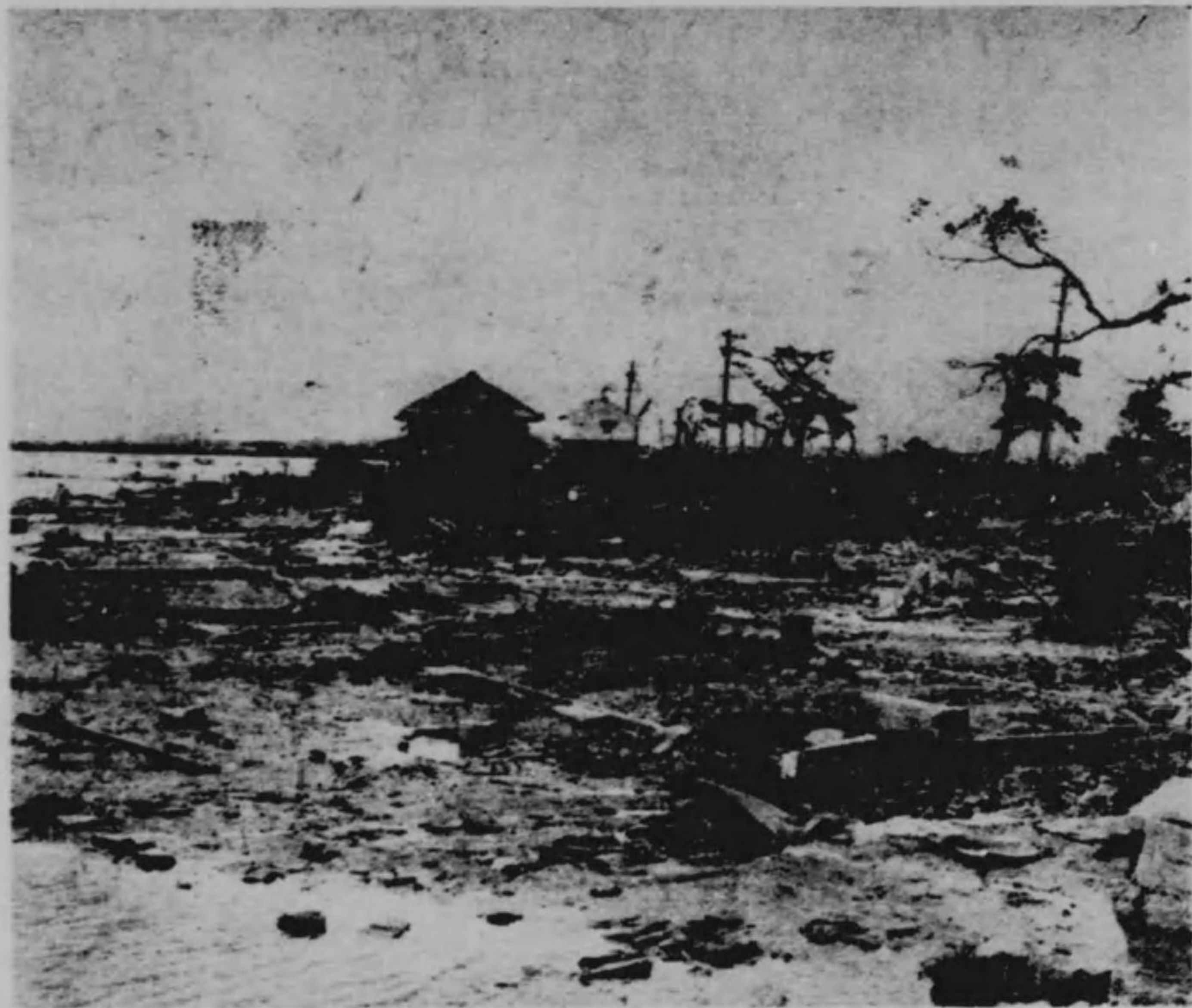
Out of nearly 300 dwellings at Nunoyamachi, Nishi Yodogawaku, Osaka city, only two houses passed safely through the storm.
