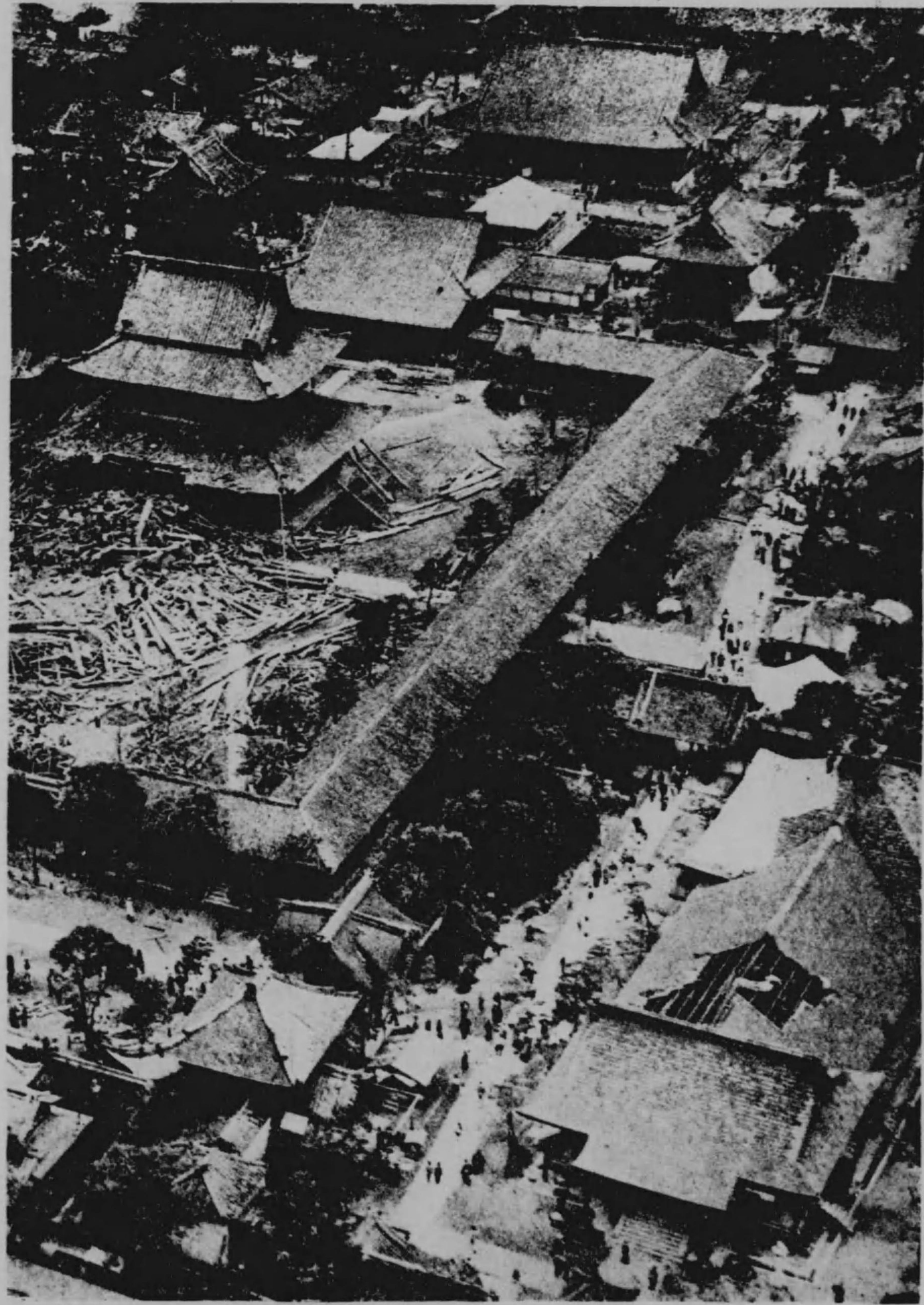
Osaka collapsed just before 8 o'clock Friday morning (21), the hall on the ground floor when the tower crashed.
