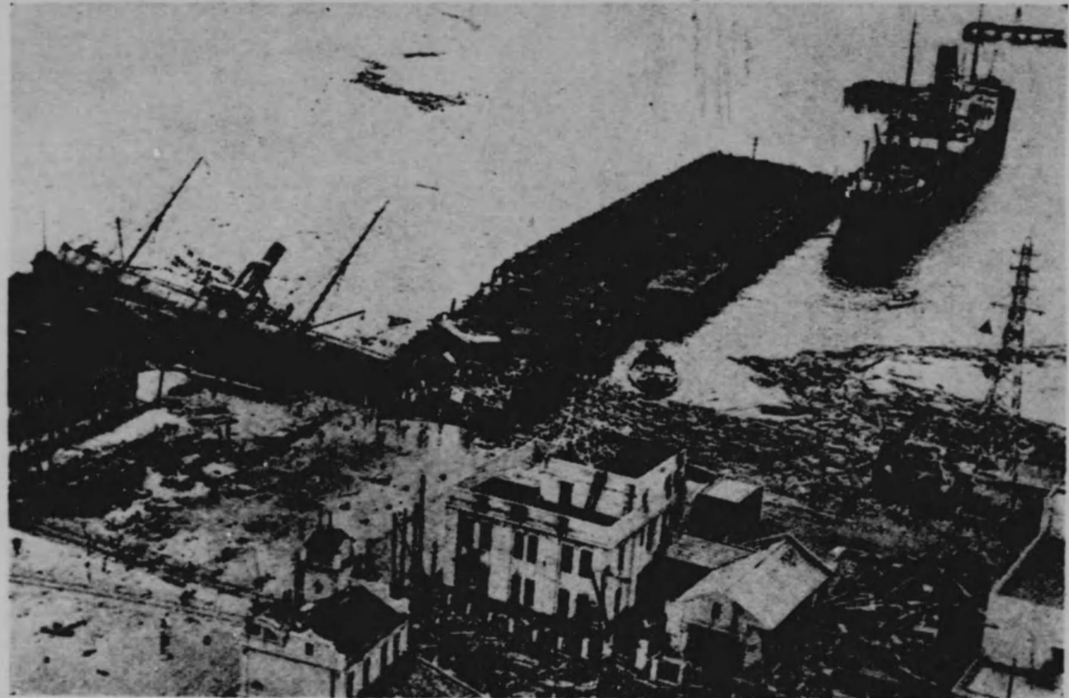
What was left of Osaka's Chikko pier.
