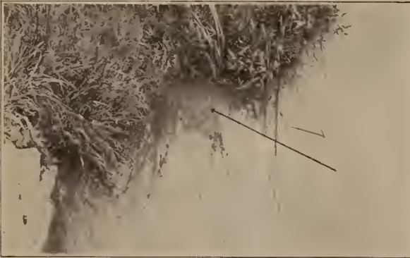
FIG. 1.—Outlet of Salisbury sewer pipe into Sampson Creek, from bridge.
