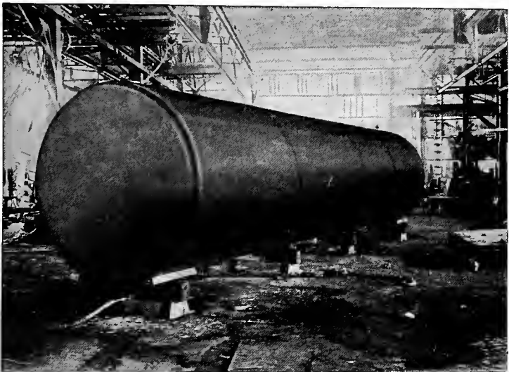
FIG. 8.—This is a Steel Tank, Made of \frac{3}{8} -inch Plate, which Measures 30 Feet Long and 8 Feet in Diameter, Fused into One Piece by the Welding Torch.
