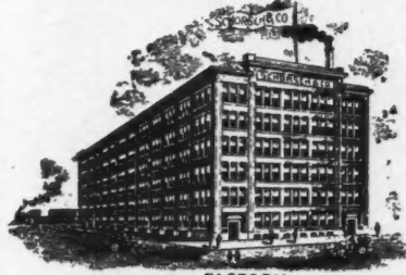
FACTORY 132 ND TO 133 RD ST & BROOK AVE
