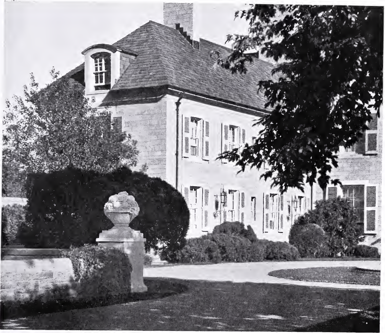
CORNER OF FORECOURT AND SERVICE WING
