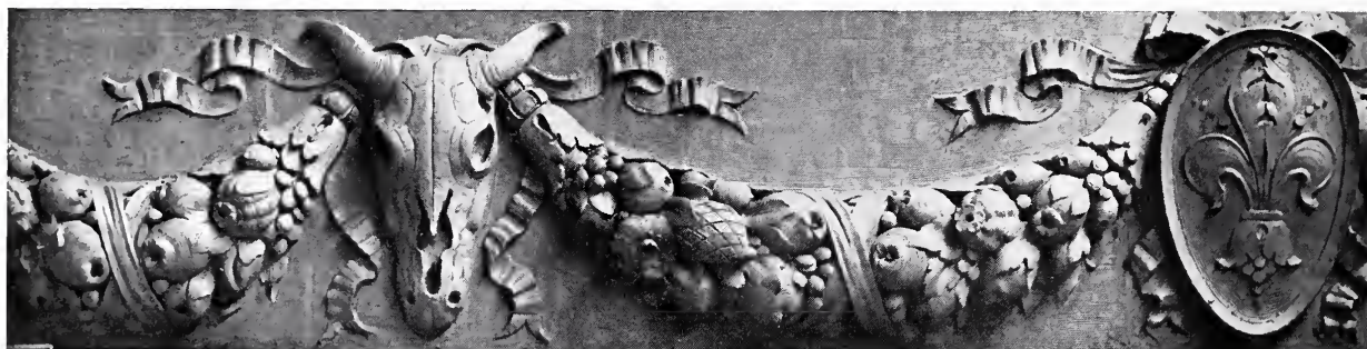
Terra Cotta Panel on Cumberland Hotel, Cumberland, Md. Frederick Webber, Architect
