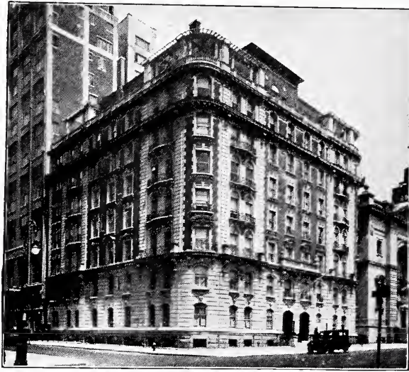
Town House Club, New York City: Starrett & Van Vleck, Architects; Crane Company, Jobbers; Fred T. Ley, Plumber
