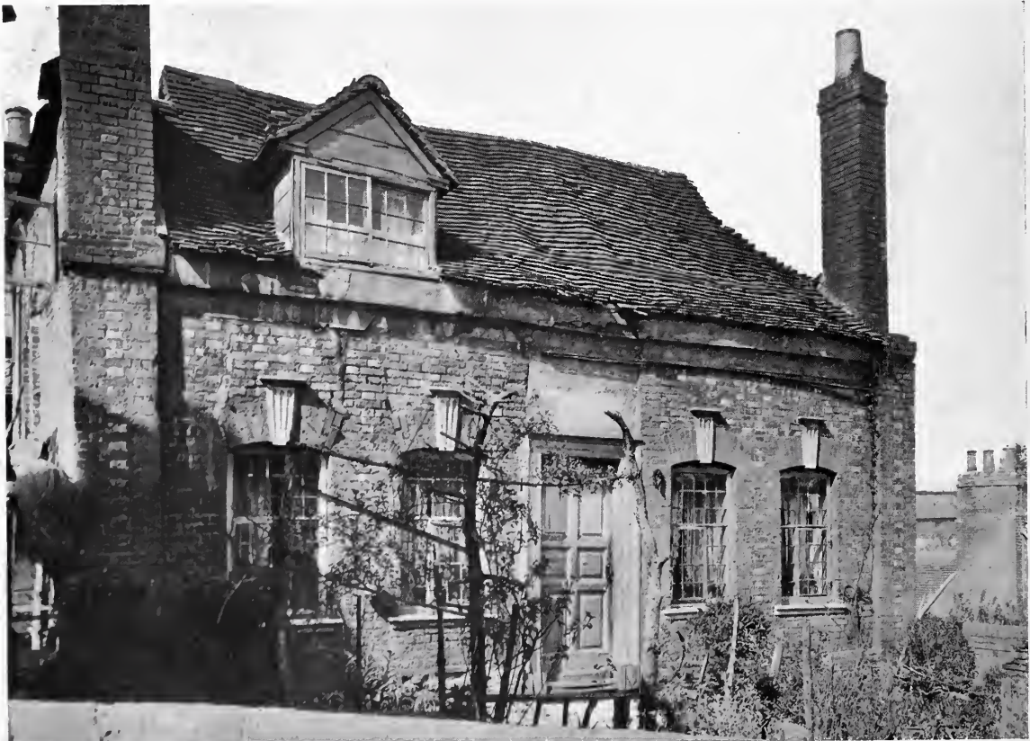
Old English Cottage of Early Georgian Character Note the leaded casements simulating double-hung windows
