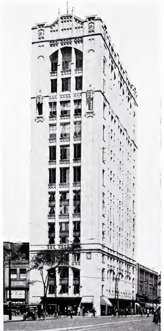
Fyfe Store Building, Detroit; Smith, Hinchman & Grylls, Architects; W. E. Wood Co., Builders. Entirely of Atlantic Terra Cotta in gray granite color and texture.
