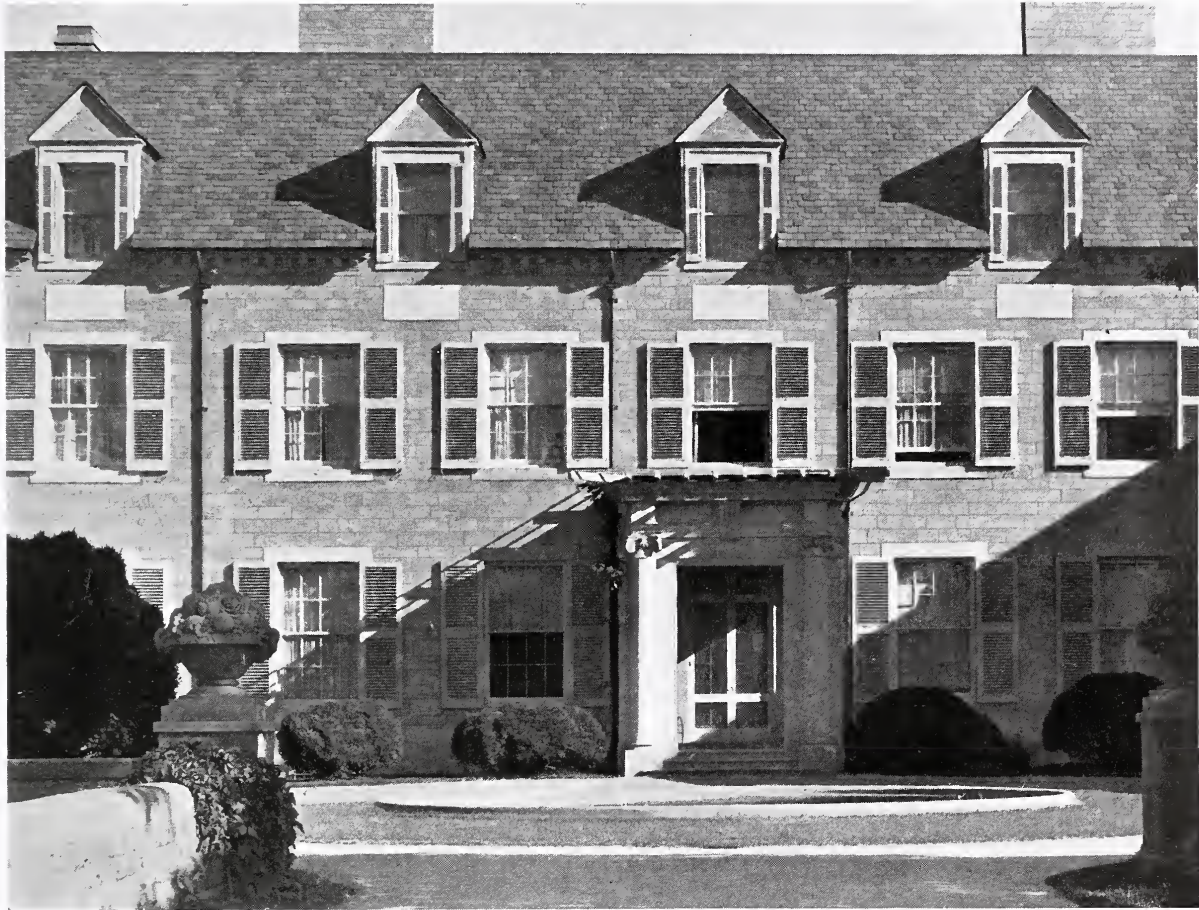
DETAIL OF ENTRANCE FACADE
