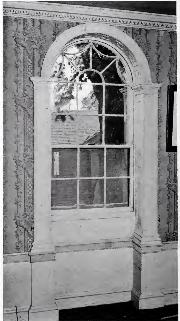
Stairway Window, Pierce-Nichols House, Salem, Mass.
