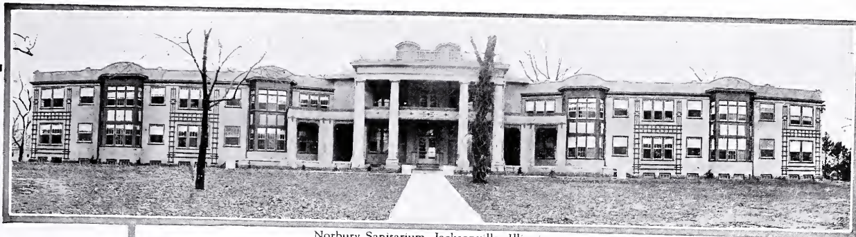
Norbury Sanitarium, Jacksonville, Illinois Jacksonville Plumbing & Heating Co., Heating Contractors C. W. Buckingham, Architect
