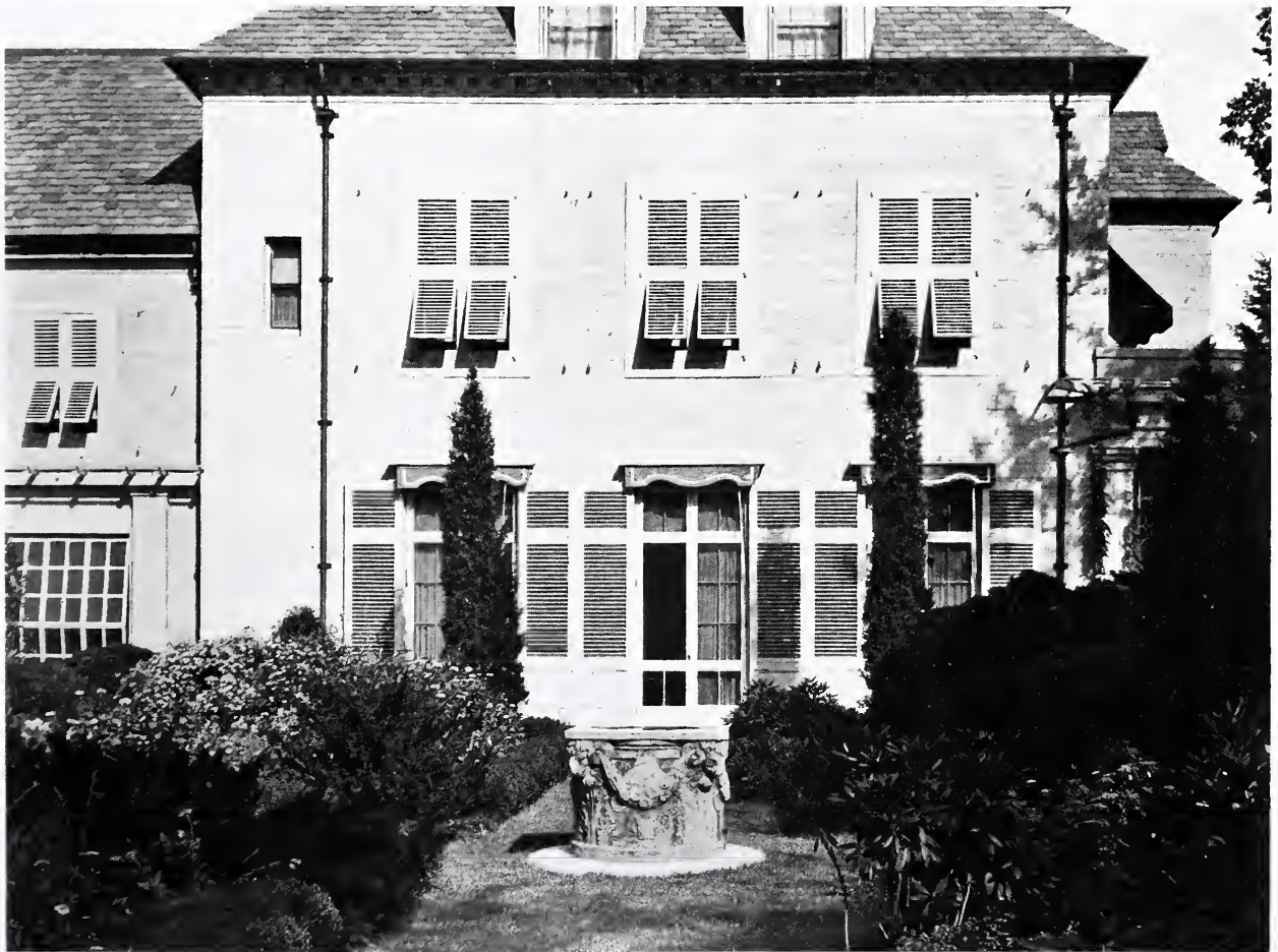
LIBRARY BAY ON WEST FACADE
