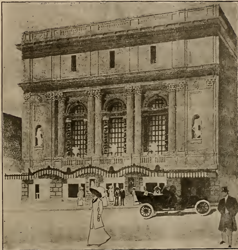
The New Columbia Theatre now in course of construction at the corner of Geary and Mason Streets.
