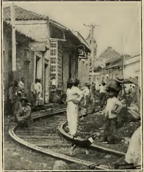
Trolley construction work in old Camaguey, corner of Avellaneda and Soledad Streets. The peculiar wooden window gratings are shown. These windows are met with but in few cities of Cuba.
