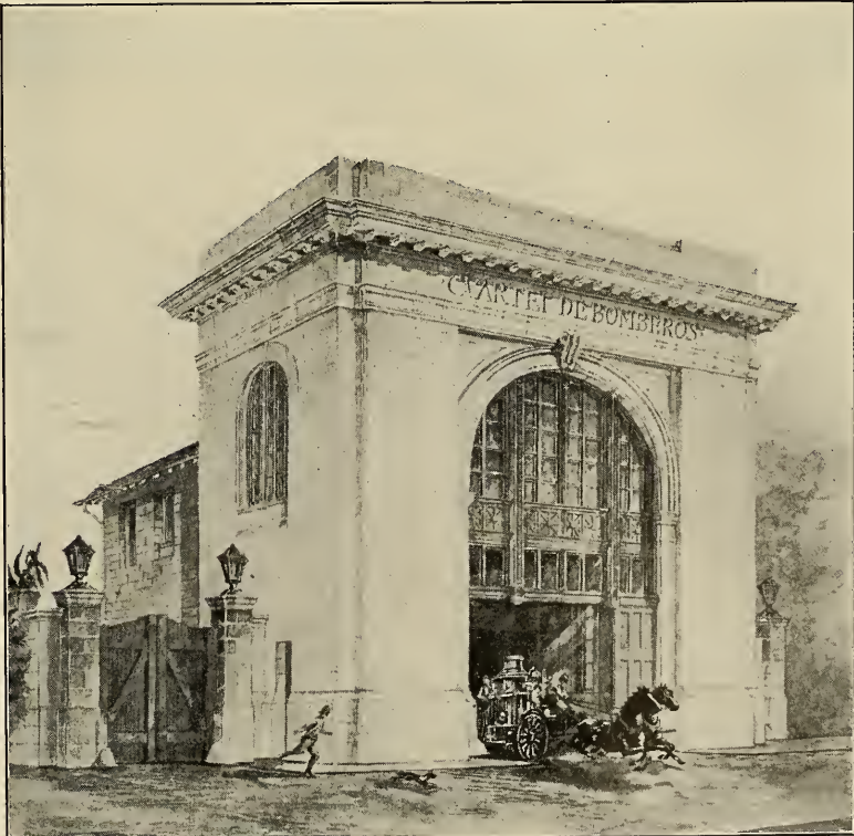
Havana's new Fire Headquarters now being built on Zulueta Street by the Department of Public Works.
