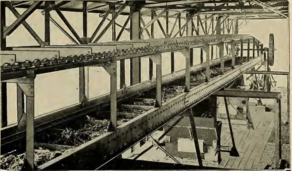
Bagasse Conveyer Over Furnaces, Showing Fuel Feeders
