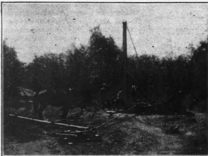
BORING IN SOFT GROUND WITH HOMEMADE DRILL
