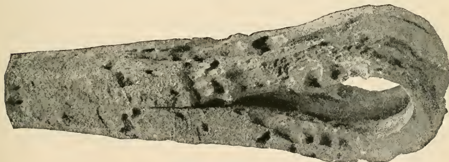
A CORRODED BRACE.
