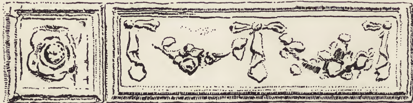
EXTERNAL PLASTER DETAILS (PARGETTING) FROM HERTS, ESSEX, AND SUFFOLK
