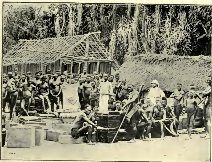
ARRIVAL OF THE REVS. F. R. ORAM AND WM. FORFEITT AT BOPOTO, TO FOUND NEW STATION, 1890. Photo: Rev. Wm. Forfeitt.
