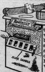
By opening the slide damper, which is placed below the fire-pot so as to secure a strong direct draft, you can have a hot fire very soon
