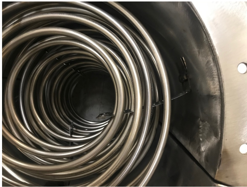
Figure 19. Brace around Heat Exchanger Coils 2
