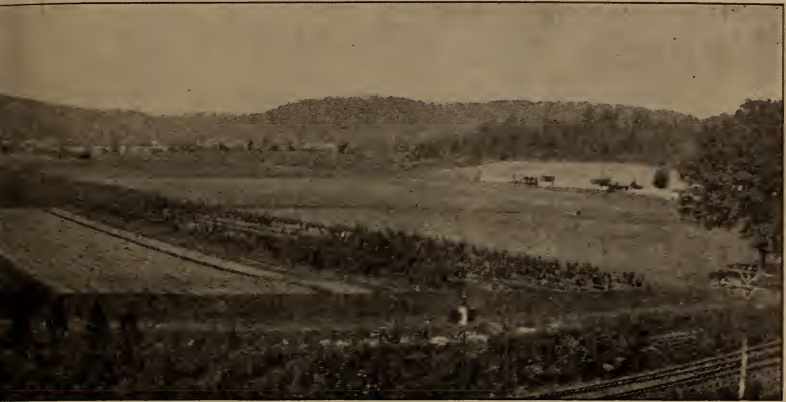
FROM TOP OF PACKING HOUSE
