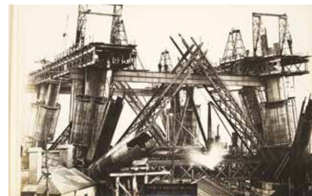
Forth Bridge, image uploaded as a part of the Resident's work
