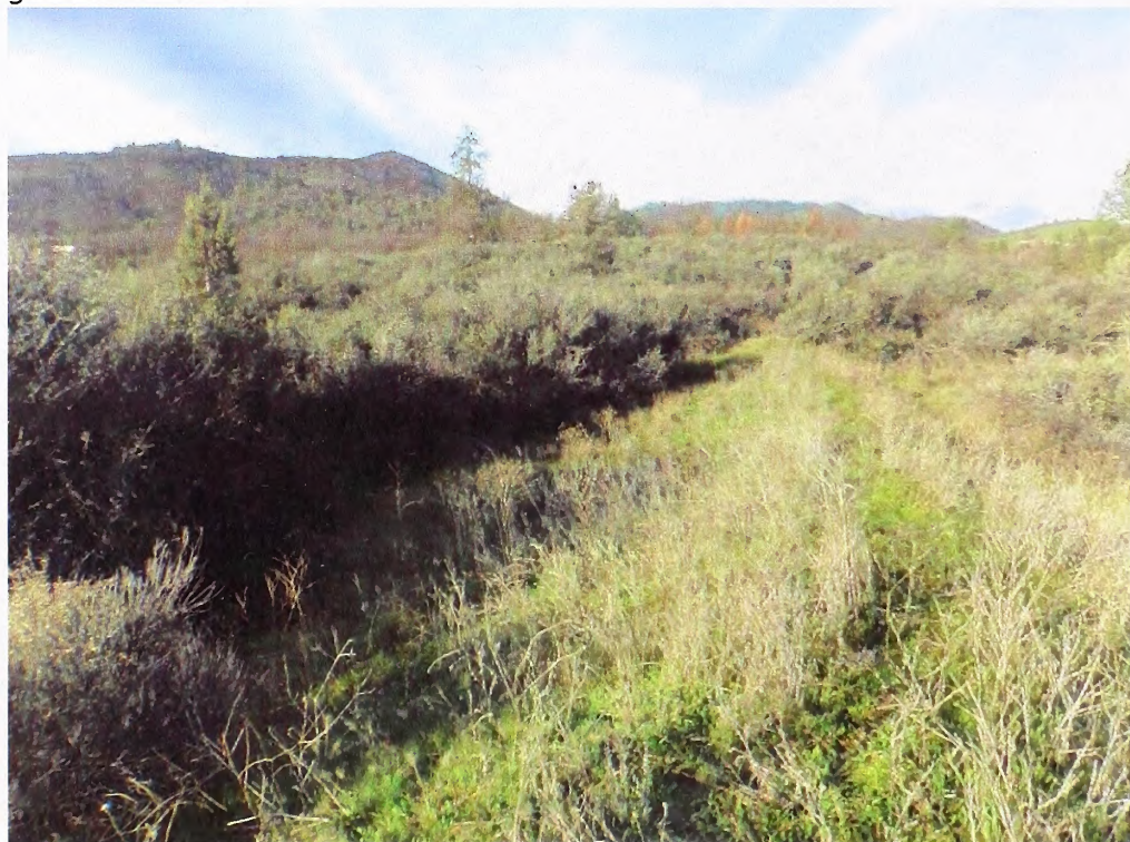
Photo 15. View west, taken from on top of east end of dam. The narrow, 25-meter long reservoir basin was formed by excavating soil from the subtle ridge crest area on the left (within the dense buckbrush) and piling it about 10-15 meters away, to the north, to form the out-curving earthen dam.
