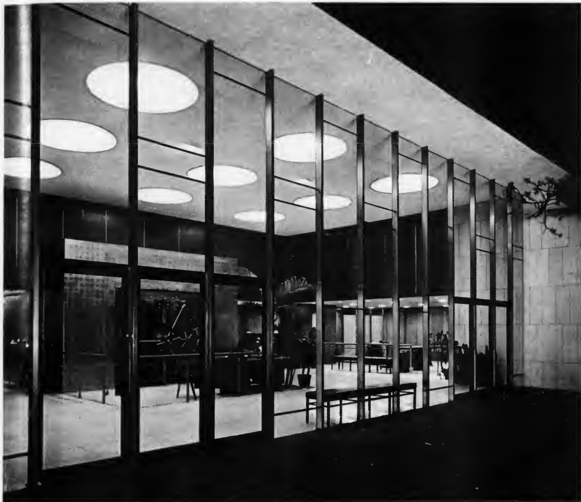
Five-foot circular diffusers of PLEXIGLAS at First National Bank of Marlin, Texas. Architect: Robert W. Maurice, AIA, Houston, Texas
