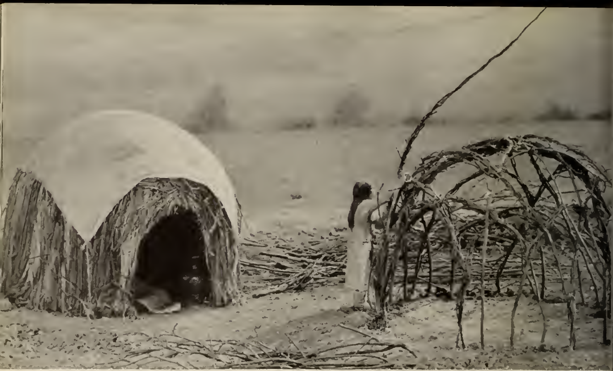
(Above) APACHE WOMAN BUILDING FRAMEWORK OF A HOUSE to be covered with thatch and rushes
