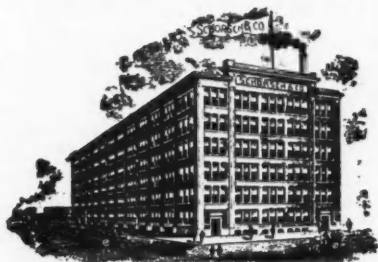
FACTORY 132 ND TO 133 RD ST. & BROOK AVE
