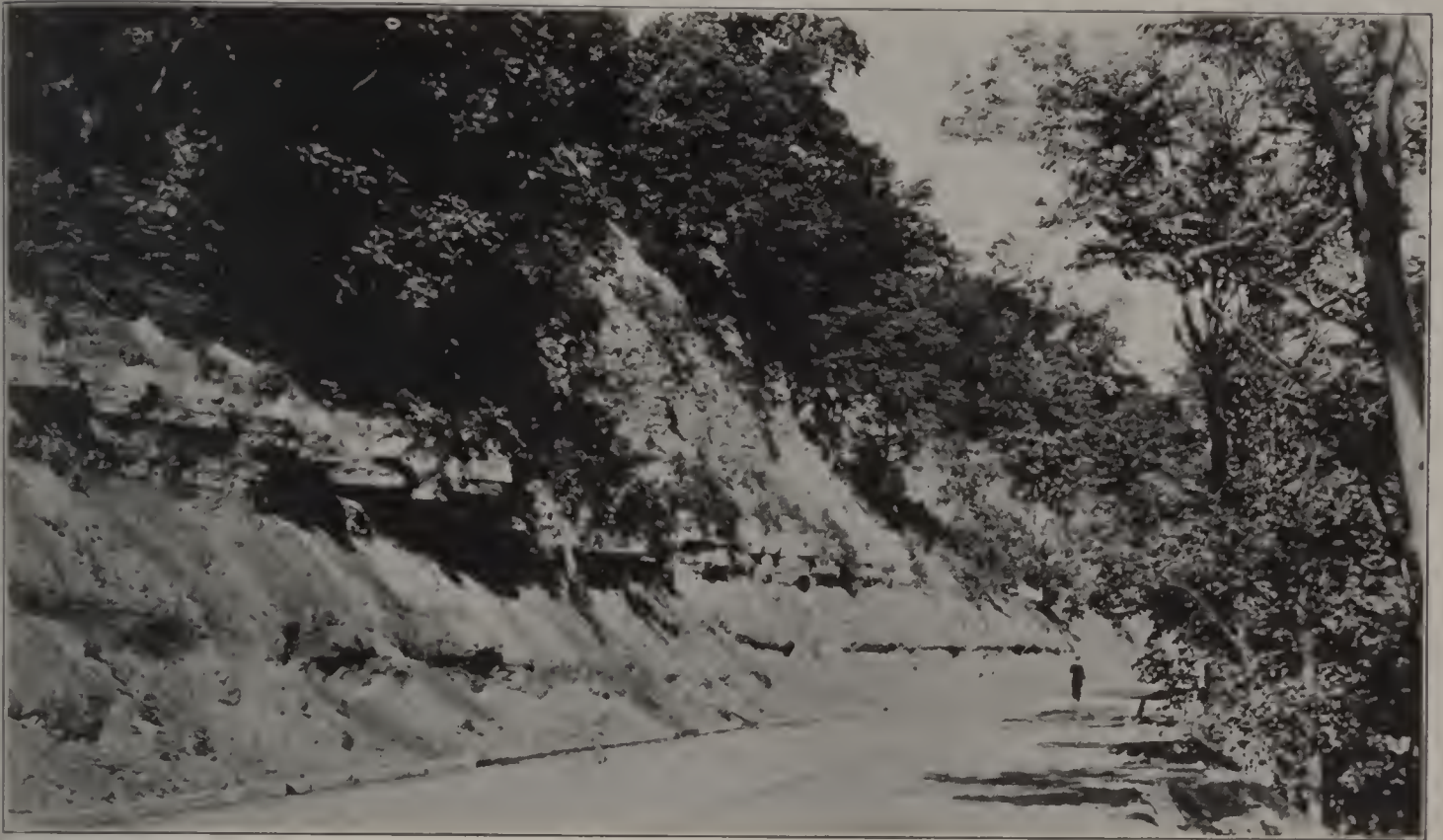
A—Projecting ledge of Putnam Hill limestone with Brookville coal below; Tionesta coal, shown by dark streak, a few feet above road. Dugway at Putnam Hill, Zanesville, Muskingum County
