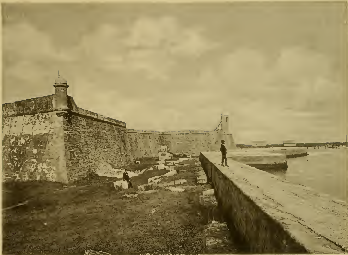
MOAT WITH HOT SHOT FURNACE, AND SEA WALL—SPANISH FORT.
