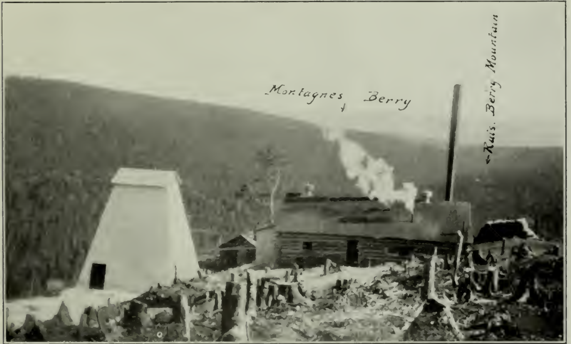
Plate III.—Shaft house and boiler plant of the Federal Zinc and Lead Co.
