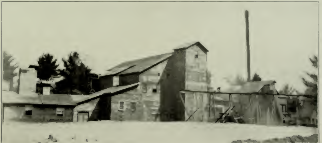
Dominion Molybdenite Co., Limited, Quyon, Que.—Concentration plant.
