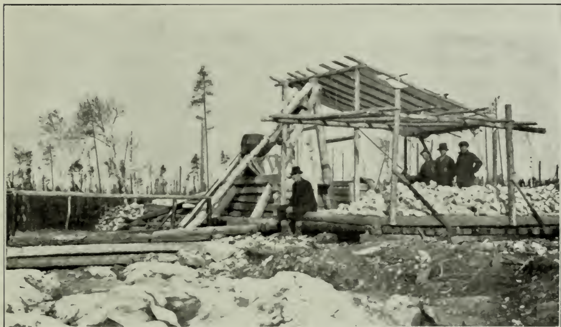
Molybdenite.—Sorting platform on Benjamin property, lots 1 and 2, range 1, township of La Corne, Abitibi.
