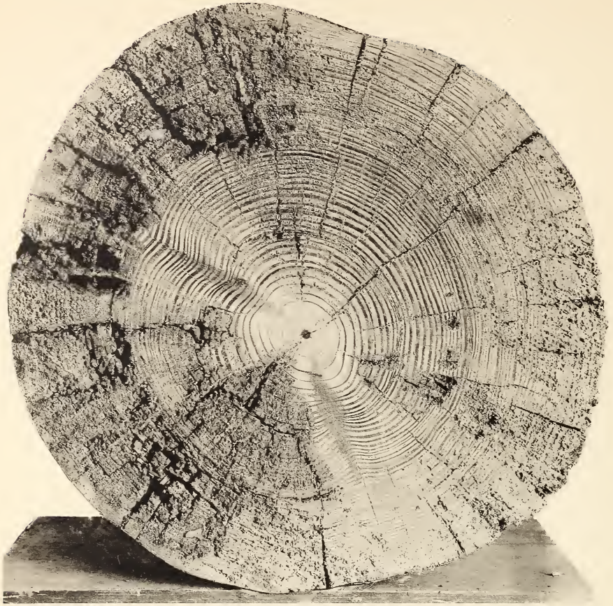
Fig. 1. Loblolly pine pile, from southern Texas, showing decay after 12 months.
