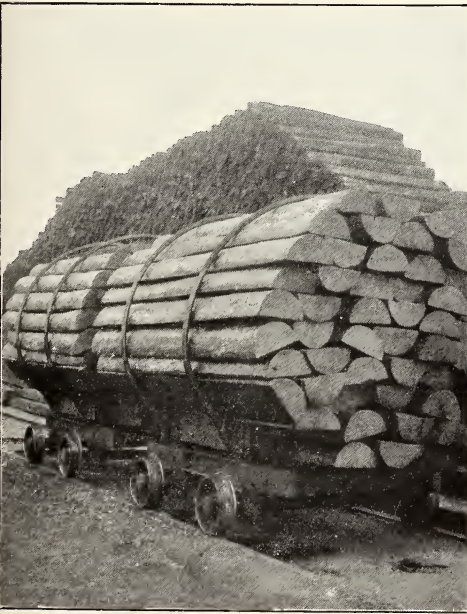
FIG. 3.—OAK TIES READY TO ENTER CYLINDER, GHENT, BELGIUM.
