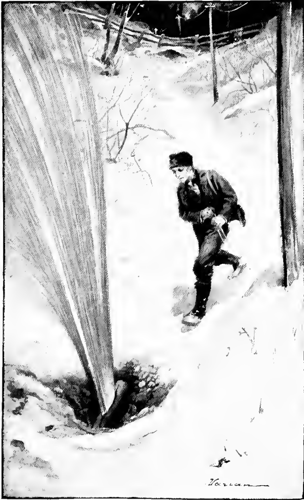
BURST IN A PIPE LINE
