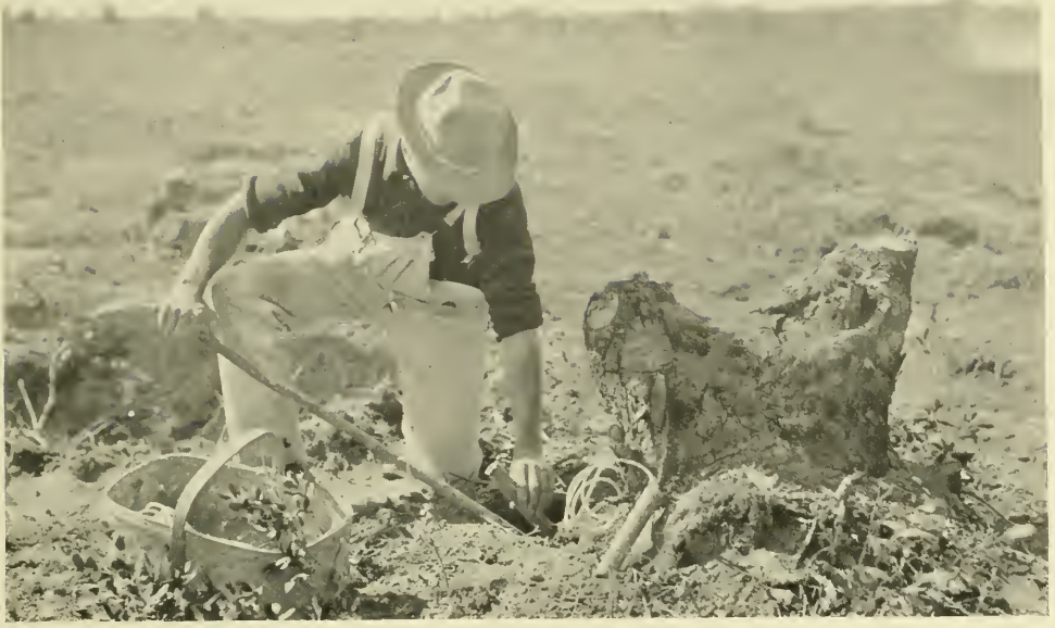
Placing one-half a pound of dynamite
