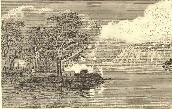
U. S. GUN-BOAT "CINCINNATI" SUNK BY THE UPPER WATER BATTERY AT VICKSBURG, MAY 27, 1863.
